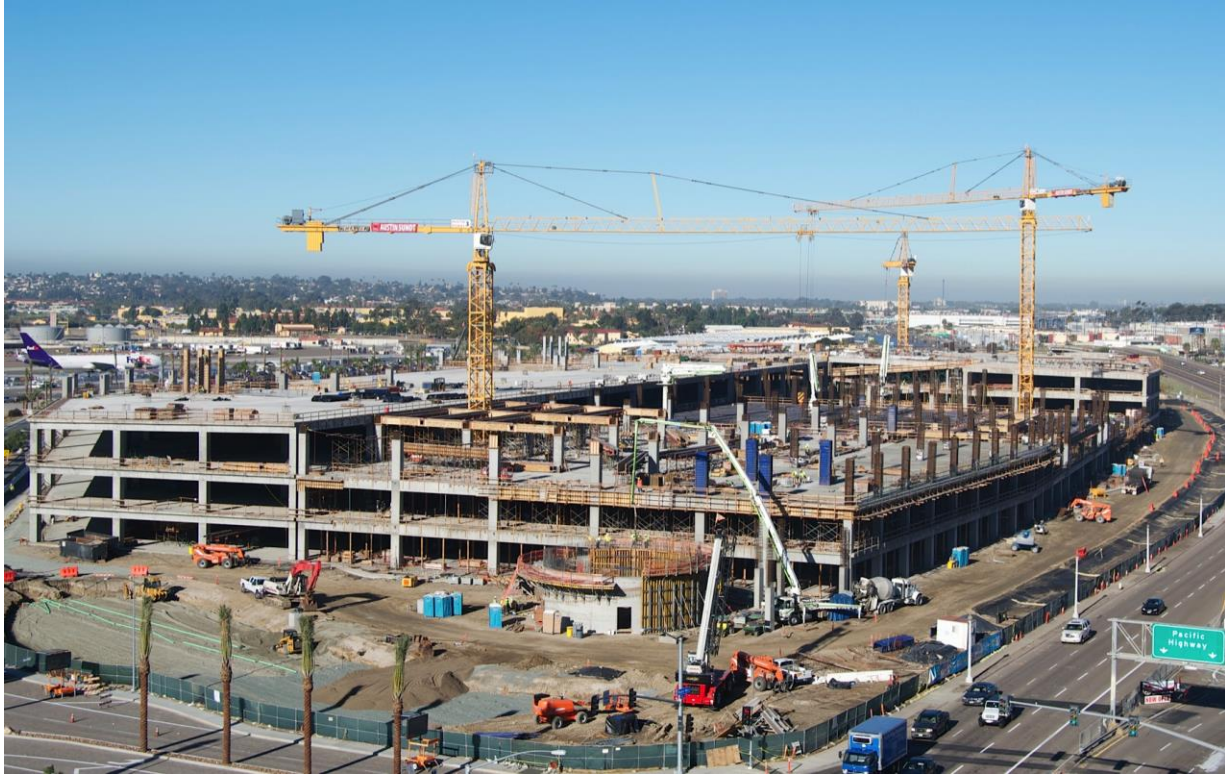
Figure 3: The "RAC" Under Construction in San Diego, CA
