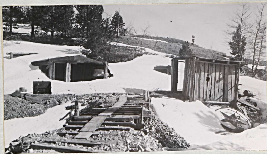
Horizontal Adit of Hidden Hand Mine in March 1951.
