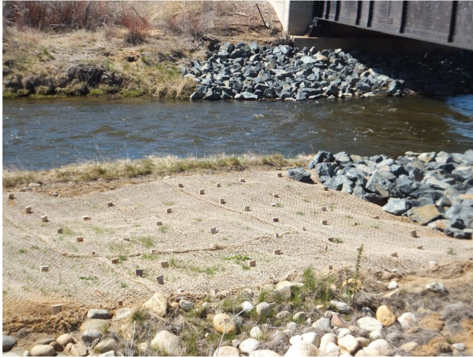
E1. Sampling area at Silver Bow Creek near the inlet to WSPOU. 5/18/2014
