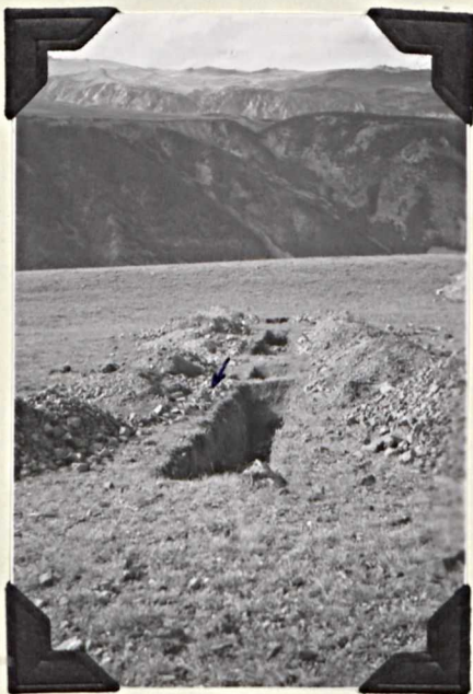
Fig. 2. View looking south toward Wyoming line from the Highline plateau. Pits and trenches contain chromite lenses and chromite broken from lenses is indicated by arrow.
