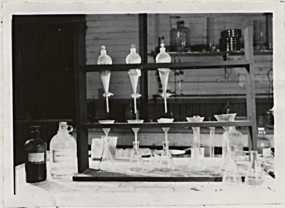
Fig. 3. The apparatus used for heavy mineral separation.
