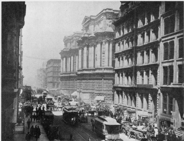
Washington Street in the Loop, looking west from Dearborn Street, circa 1893 (From Chicago 1892 , Chicago Historical Society).
