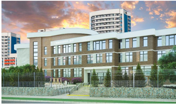
Figure 2.1. Main façade view
