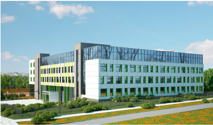
Figure 1.1. Main façade view with continuous glazing and the increased height of the first floor
