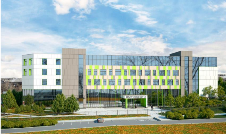
Figure 1.3. Main façade view with continuous glazing and the increased height of the first floor
