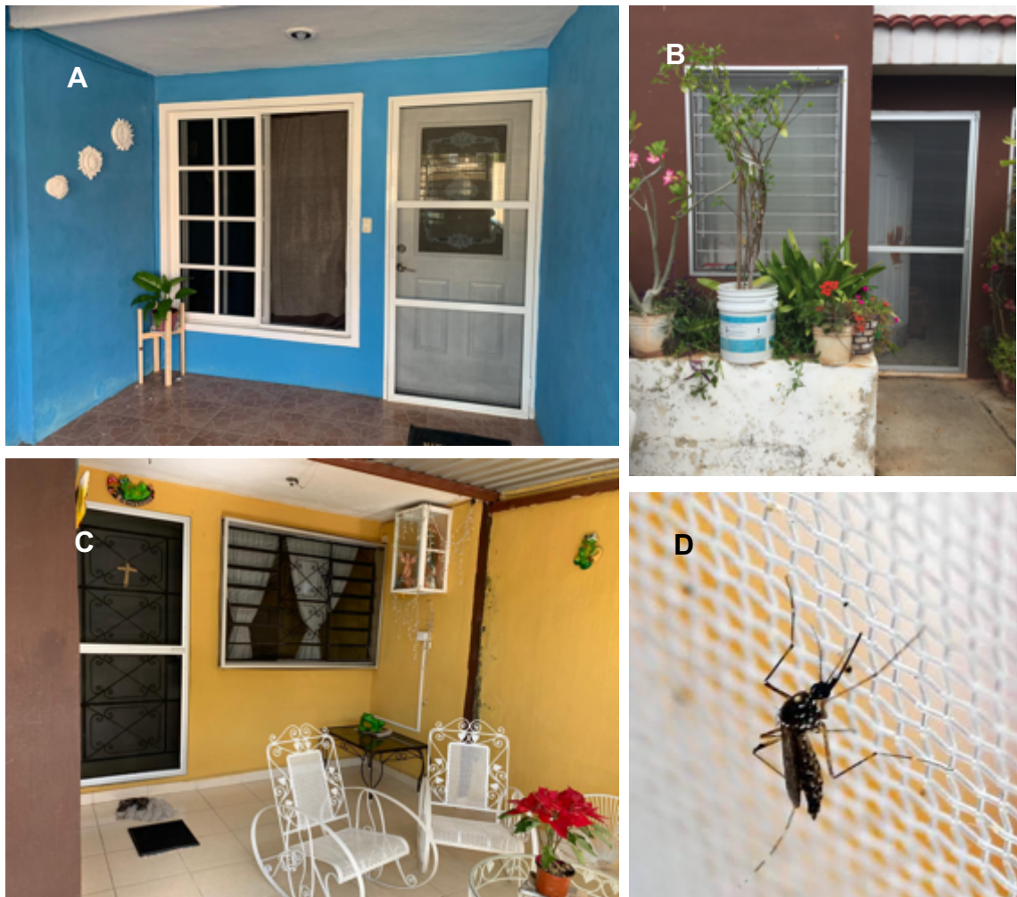
Figure 2. A-C: House screening -with regular netting mounted on aluminium frames- installed on doors and windows of houses at Merida, Mexico. D: Female Aedes aegypti standing on a screen.
