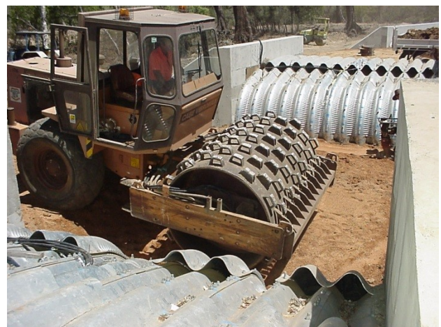
Fig. 6: Compaction of the backfill soil
