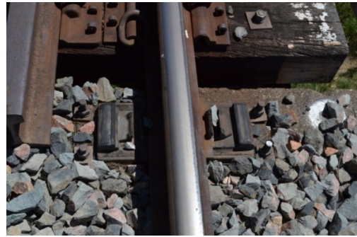
Fig. 10 The ALT.1 Delkor plate is installed on the abutment / ballast log
