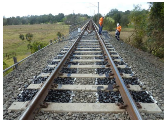
Fig. 15 Area for ballast glue at the bridge end
