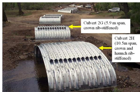
Fig. 4: The Mandalee Super-Cor rib reinforced corrugated steel box culvert structures, Queensland, Australia, 2002 (Ingal Civil Products)
