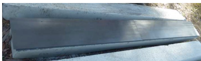
Fig. 9: The under sleeper pads are glued to the sleeper underneath
