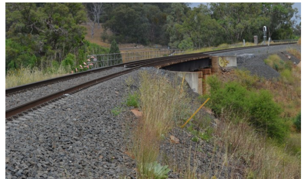
Fig.2 Transition between embankment and steel girder bridge
