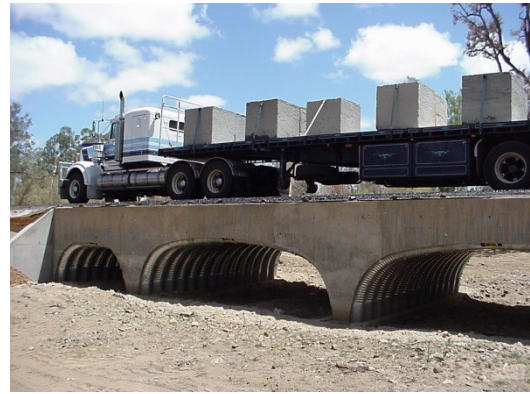
Fig.15: Live load testing on the buried culverts
