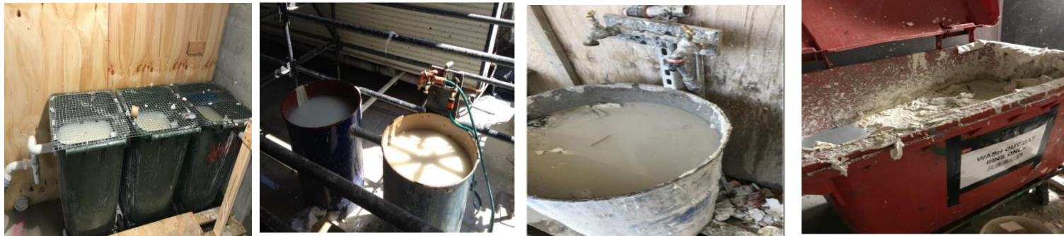
Figure 4.3 : Other examples of drum style washout systems used on-site handled by large and medium-size builders
