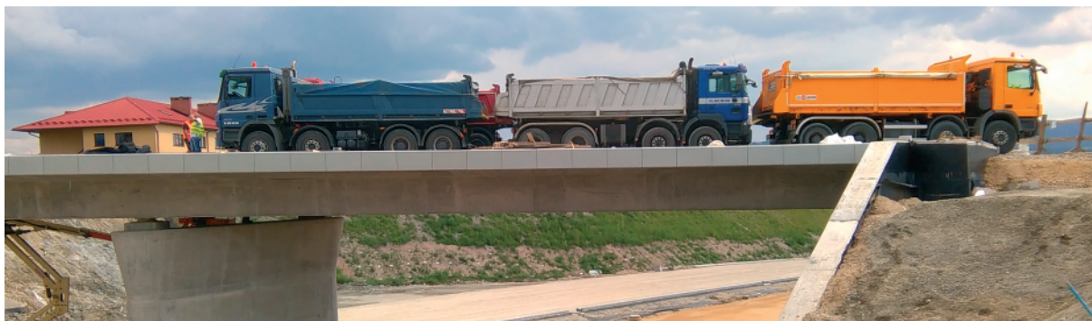
Figure 3. Exemplary typical bridge under test loading
