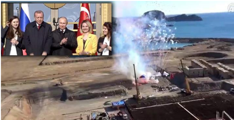
Figure 5. Foundation of Akkuyu Nuclear Power Plant [57].
