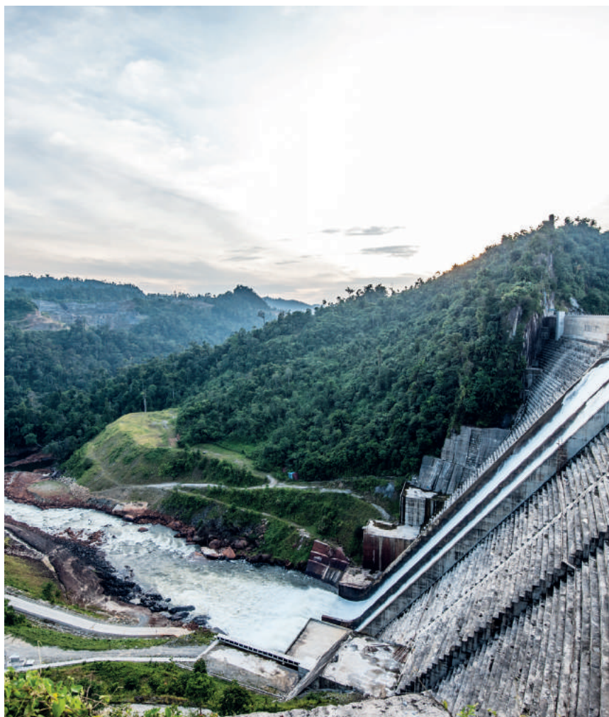
The 944MW Murum Hydroelectric Plant.
