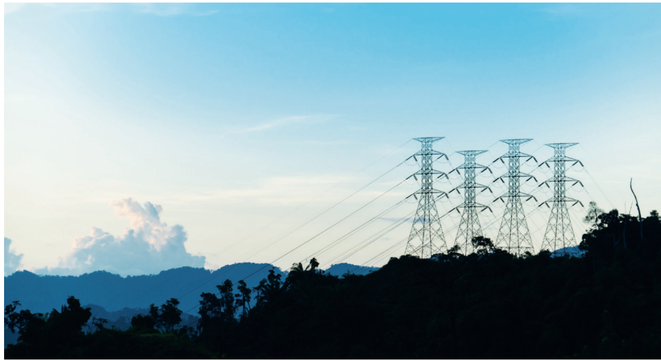
Sharing renewable energy resources with regional neighbours: In 2016, Sarawak began exporting energy to West Kalimantan in Indonesia through a 120km 275kV double circuit transmission line stretching from Mambong in Sarawak to Bengkayang, West Kalimantan.
