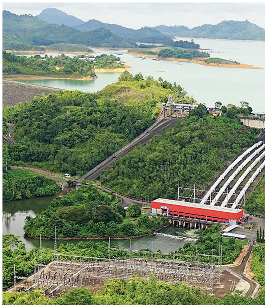
Operating for more than 30 years, the 108MW Batang Ai continues to create value and sustainability.
