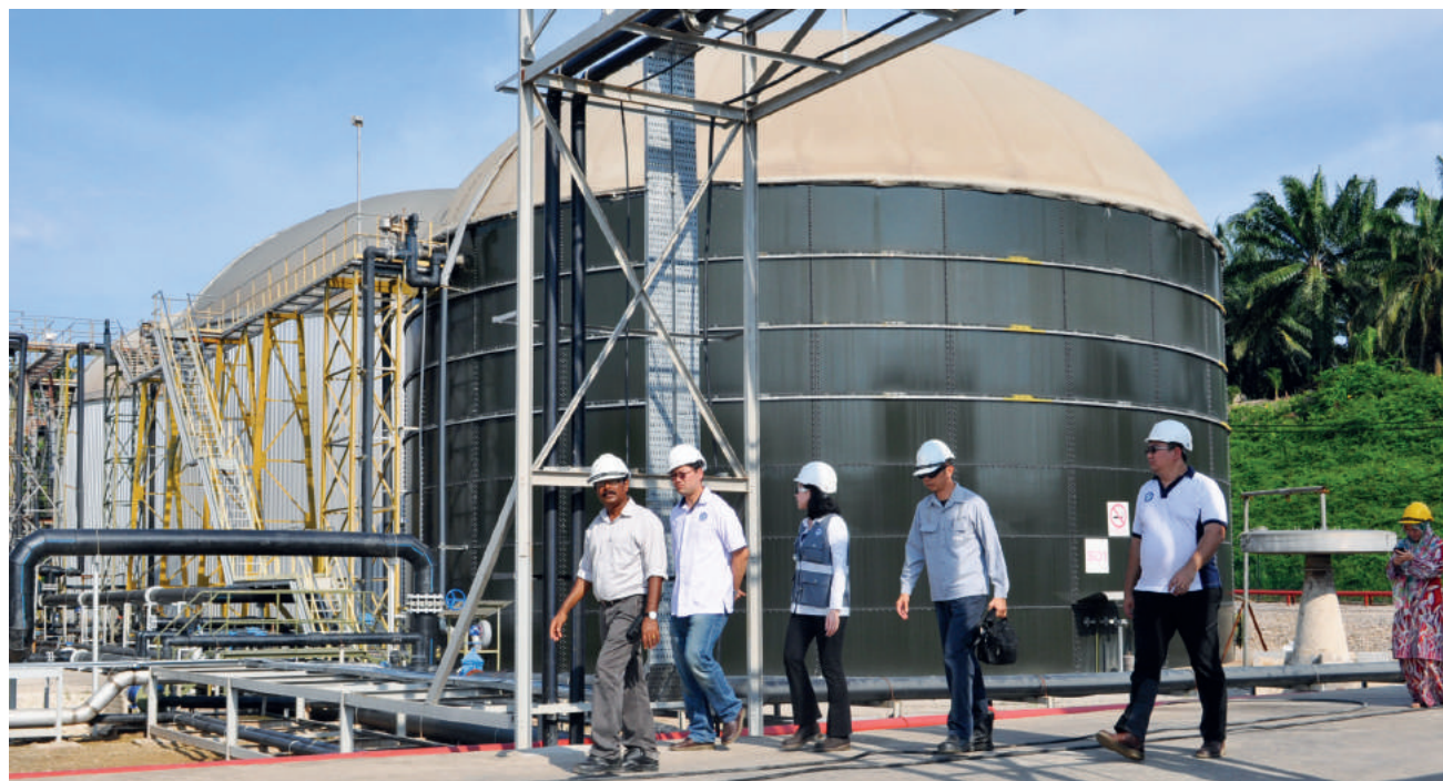
SEDA personnel monitoring a 4 MW biogas plant owned by Mistral Engineering Sdn Bhd in Sandakan, Sabah.
