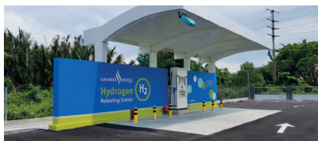
Southeast Asia's first integrated hydrogen production plant and refuelling station in Kuching.
