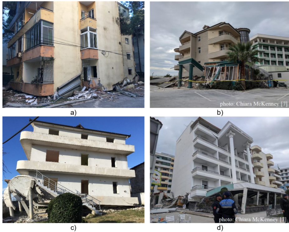
Figure 3. Examples of building collapses due to “soft storey” effect in the November 26, 2019
