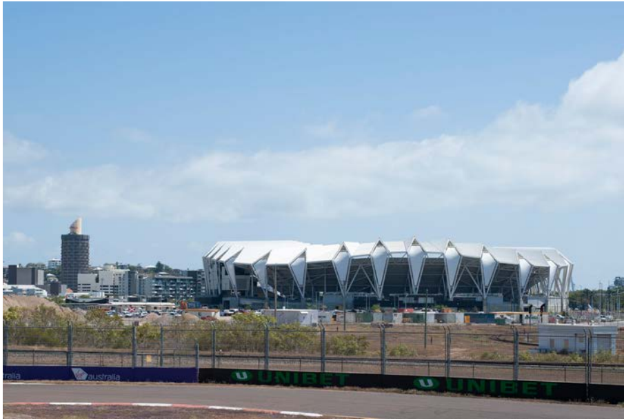
Urban Construct Boundary St #1 2019
