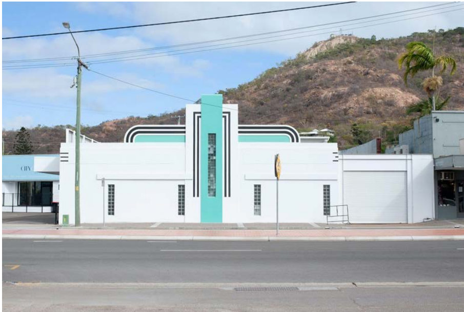
Urban Construct Flinders St #1 2019
