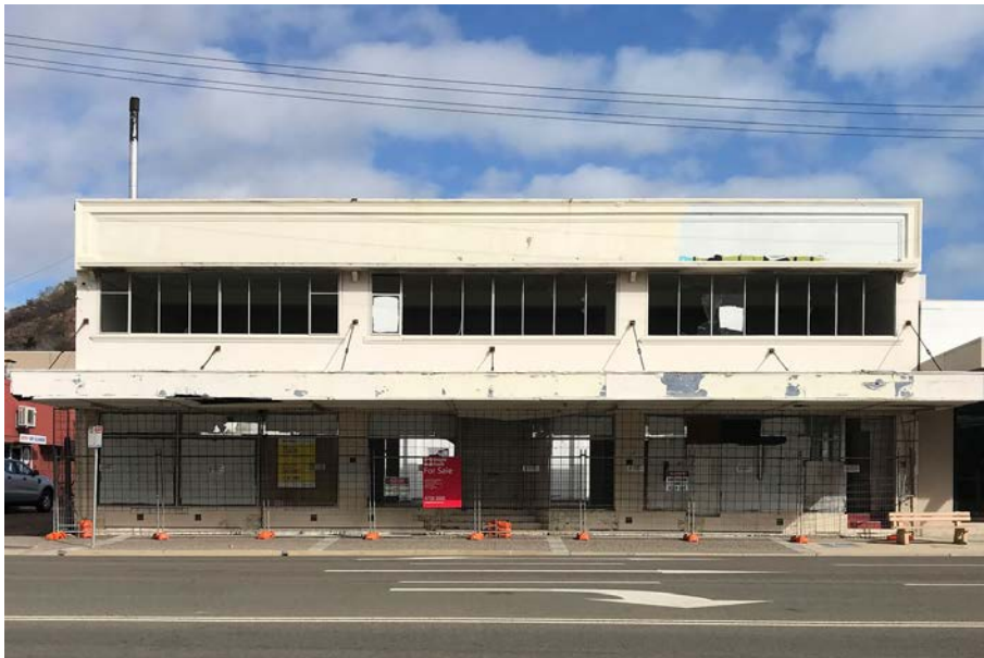
Urban Construct Flinders St #2 2019
