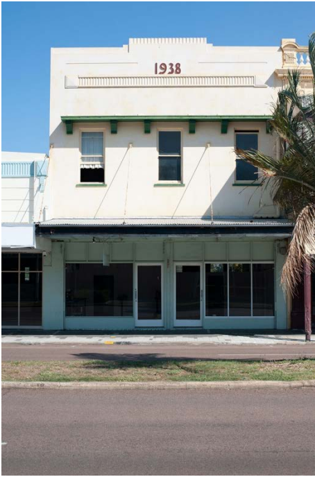
Urban Construct Flinders St #3 2019
