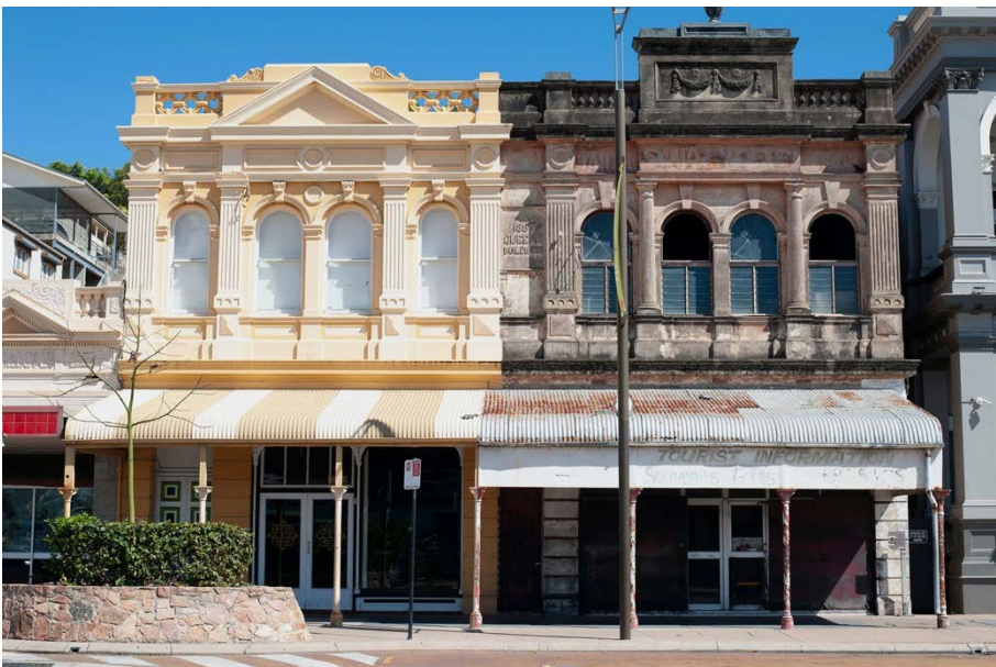
Urban Construct Flinders St #5 2019
