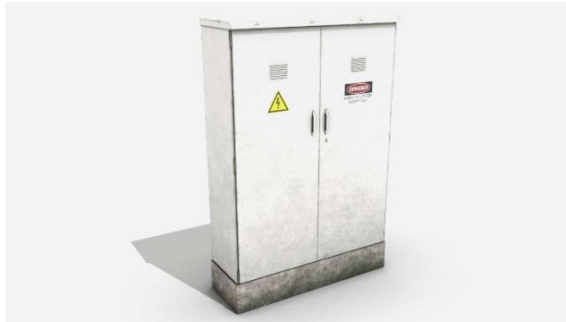
Figure 4.2 – street electrical cabinets
