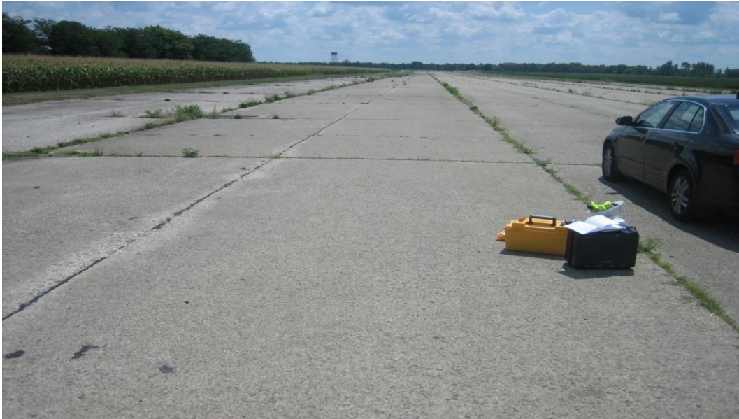
Figure 5.22 View of Rantoul Airport slab to be tested
