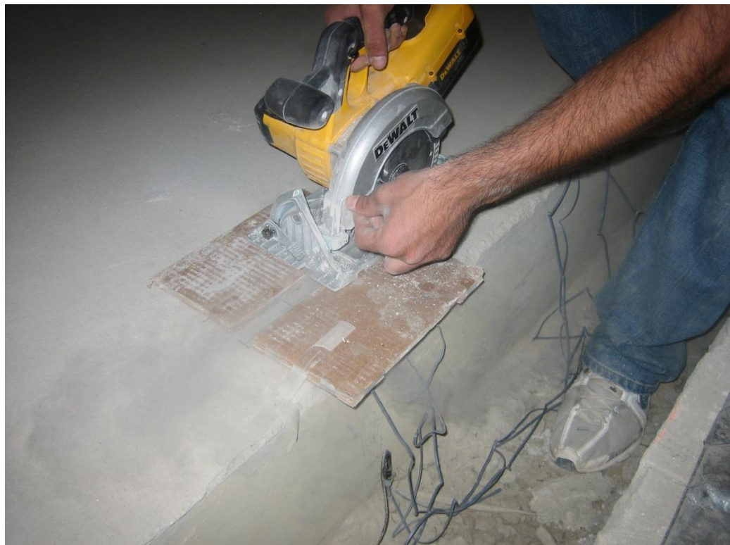
Figure 4.38 Revised notching geometry for test B1. Note the battery powered circular saw in use.
