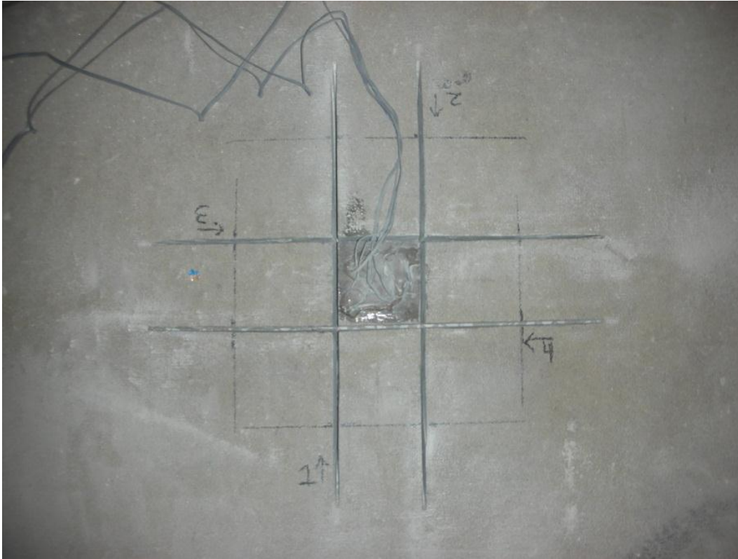
Figure 2.4 Four saw notches surrounding a rosette of 30mm strain gages cut to a depth of 1.0 inch
