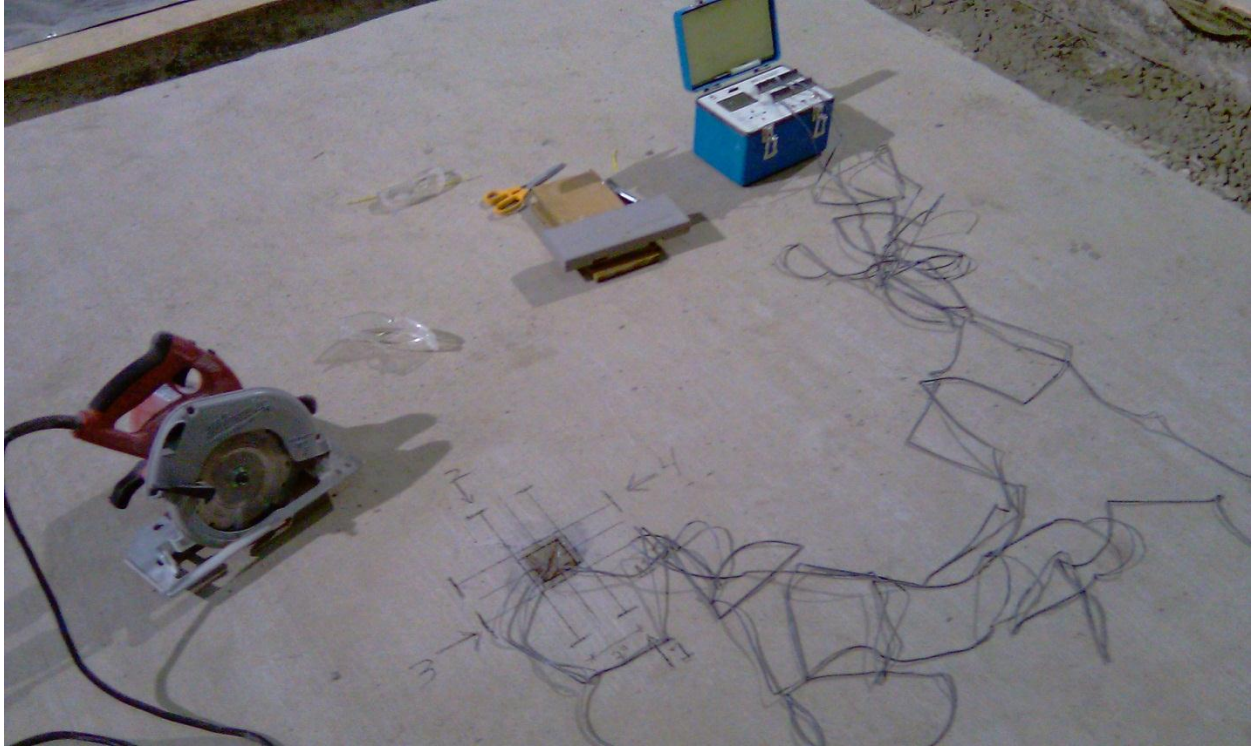
Figure 4.27 Testing of A1, typical testing layout
