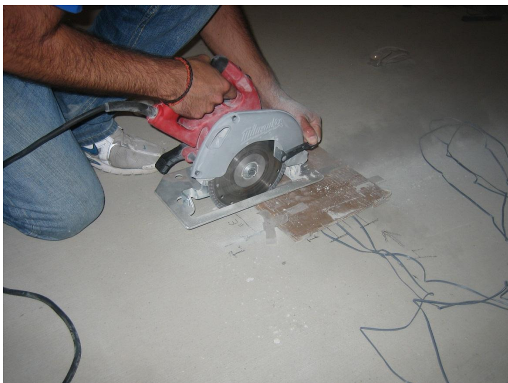
Figure 4.36 Lowering the saw blade at one end of the guide line
