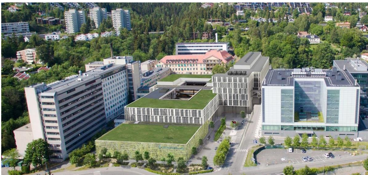
Figure 5.3-1: Digital illustration of the building design of the four new building wings at the Radium Hospital (Helse Sør-Øst, 2021).
