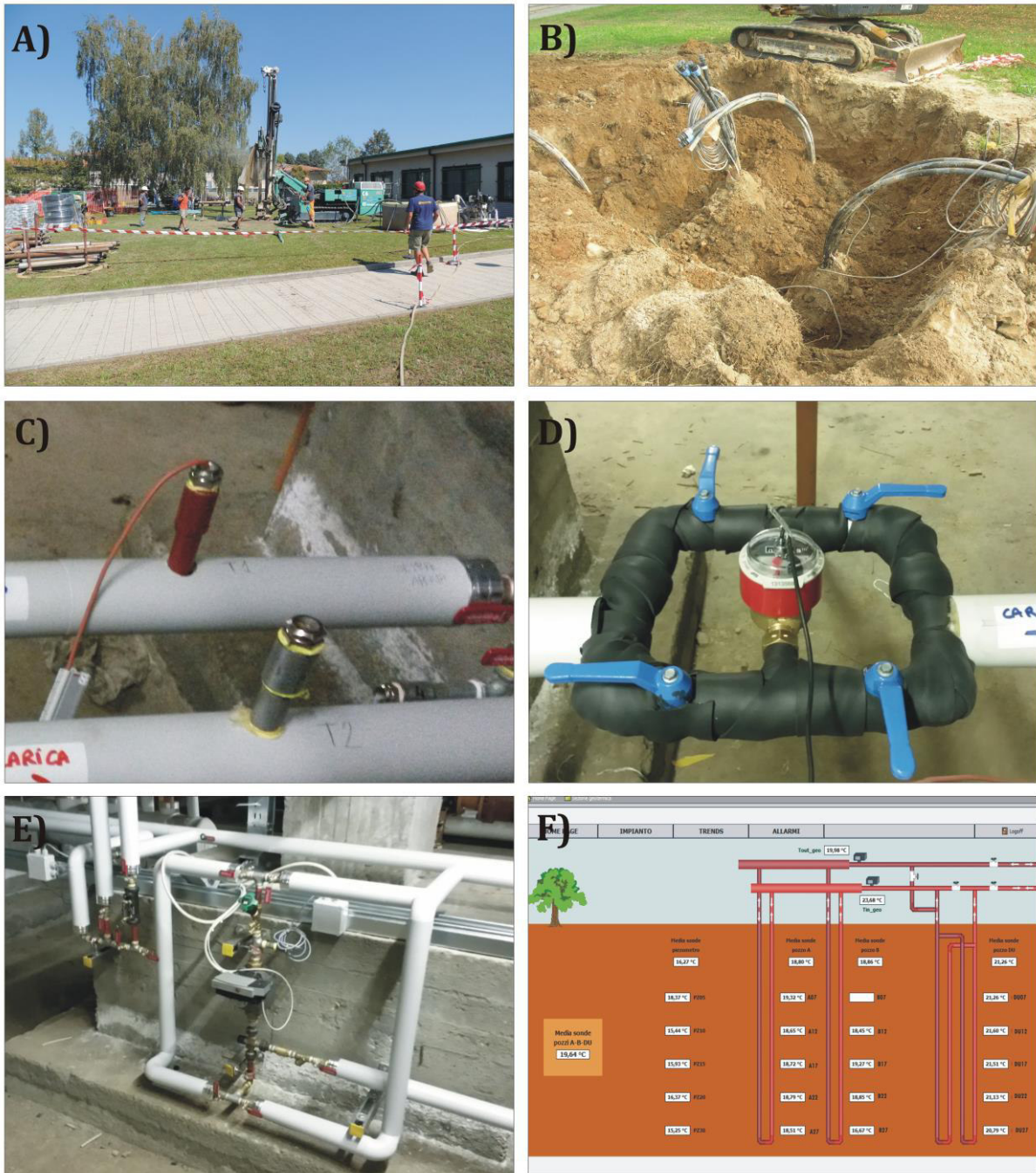
Fig. 8 – Pictures of the living lab. Drilling activity in front of the Topography department (A-B); temperature sensors placed throughout the circuit (C); ultrasonic flow meter (D); hydraulic circuit of the plant (E); underground section of the remote control system (F).
