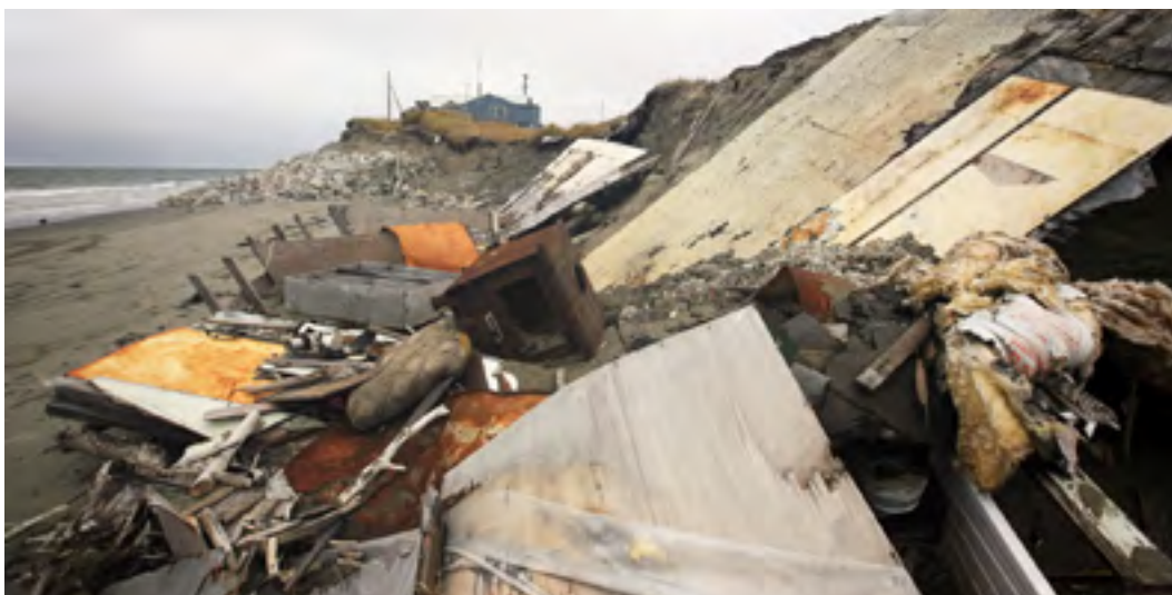
Houses collapsing due to coastal erosion in Shishmaref, Alaska. Lawrence Hislop / GRID-Arendal
