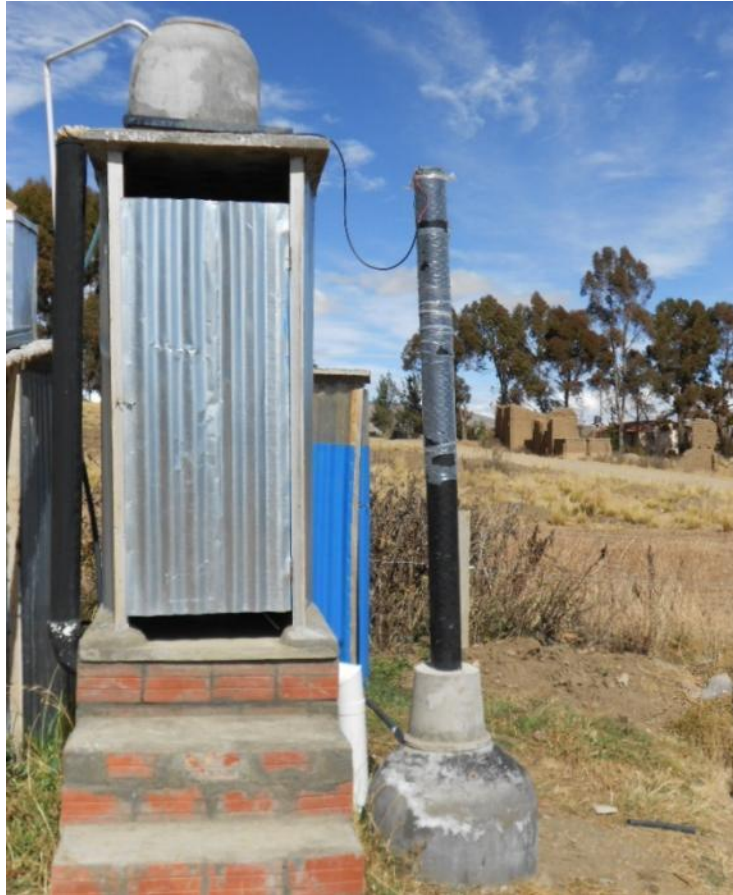
EMAS latrine for urban applications with odour filtration unit attached
