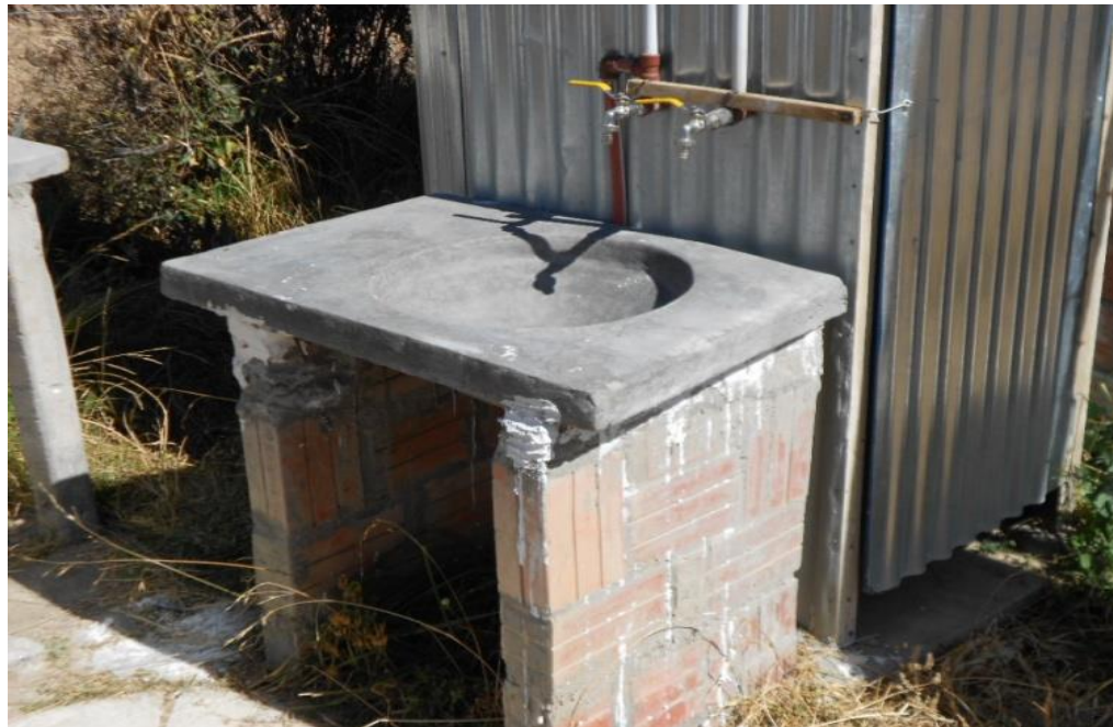
Ferrocement Sink fitted to EMAS shower house
