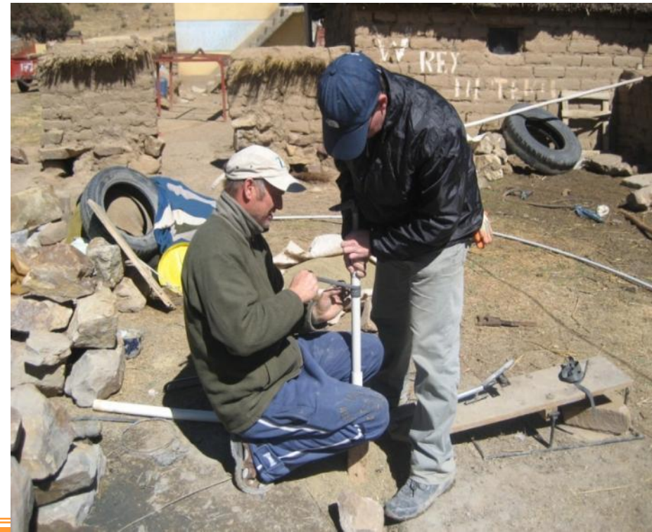
Fitting the standard EMAS handpump to family well in Corapata
