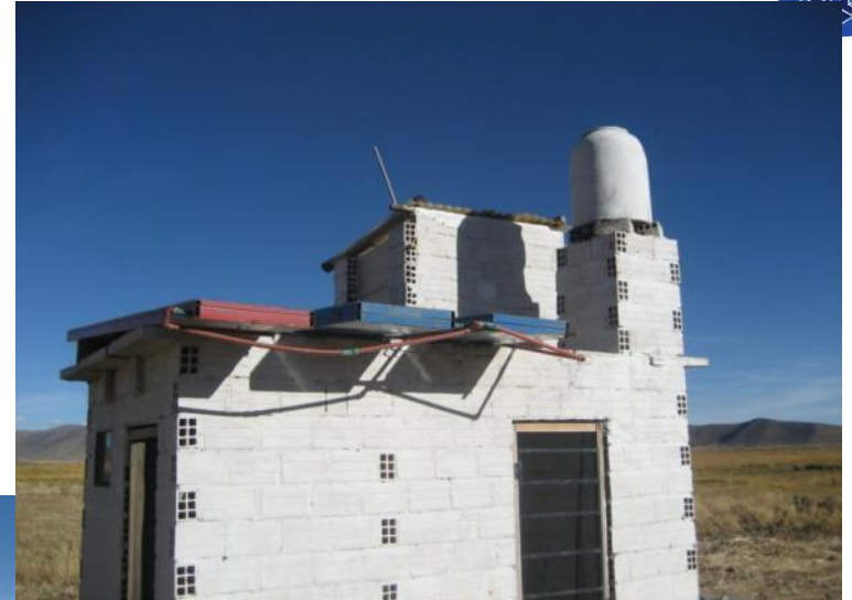
Community Wash House with solar water heaters
