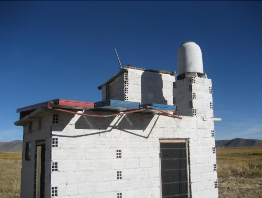
Teach nócháin pobail le Téitheoir gréine don uisce Community Wash House with solar water heaters
