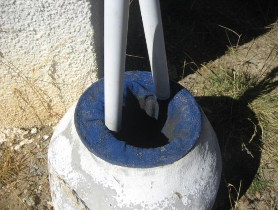
Rainwater filter comprising fleece material
