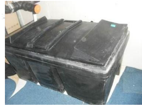
3. RWH HEADER TANK
