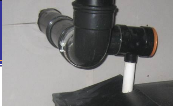
2. RWH SYSTEM OVERFLOW & FILTER
