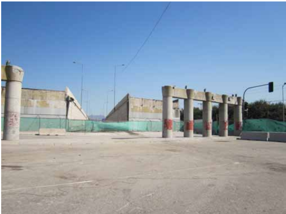
Figure 3.41 Mechanically stabilized earth, bridge ring 2, Miraflores Bridge, Santiago, April 13, 2010 (-33.394269°,-70.769402°)
