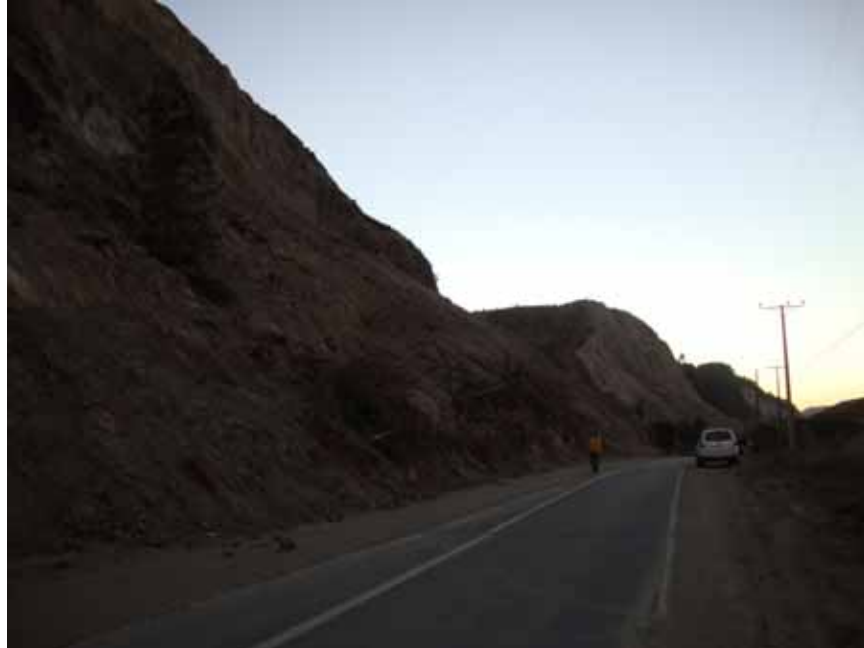
Figure 3.4 Arauco landslides/coastal bluff features, note linear feature in the road showing a vertical offset, April 14, 2010
