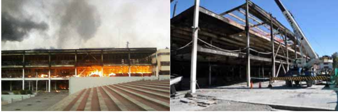
Figure 4.13 Fire in the Chemistry Building after the earthquake and the demolishing process
