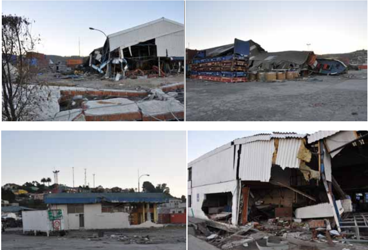
Figure 4.24 Damaged buildings of the Talcahuano port
