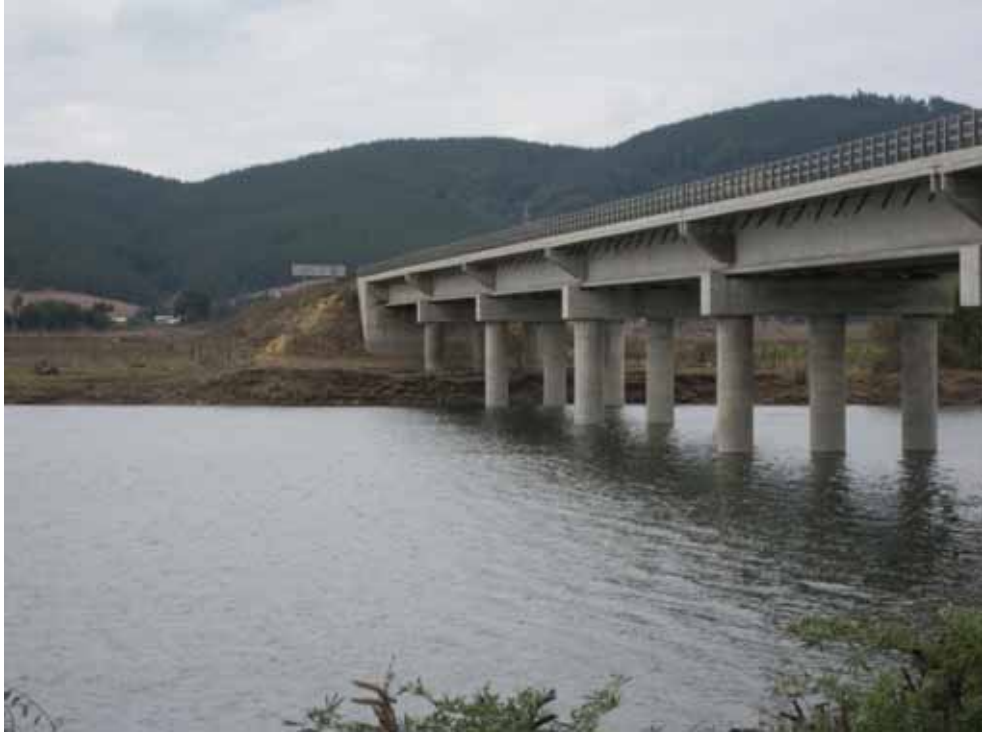
Figure 3.28 Lateral spreading on the north end of the bridge, Puente Mataquito, April 16, 2010 (-35.050712°,-72.162258°)
