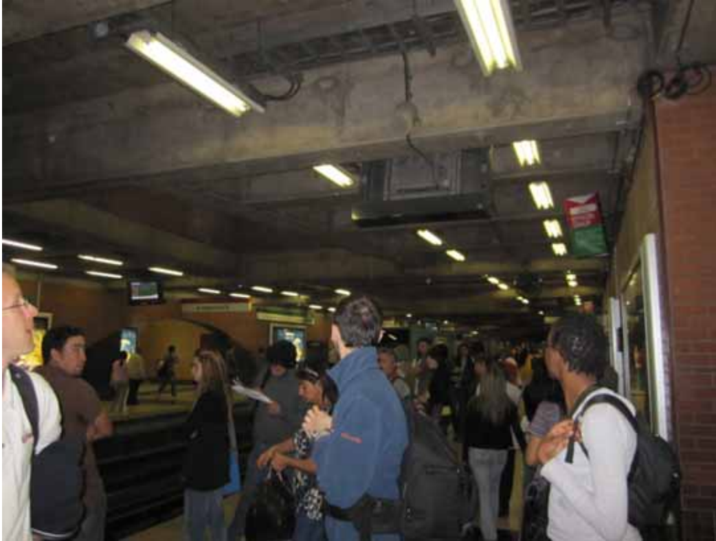
Figure 3.38 Santiago Metro, Baquedano Station, April 12, 2010
