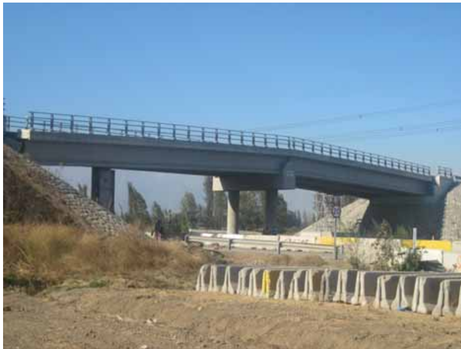
Figure 4.82 Case study overpass bridge crossing Route 5
