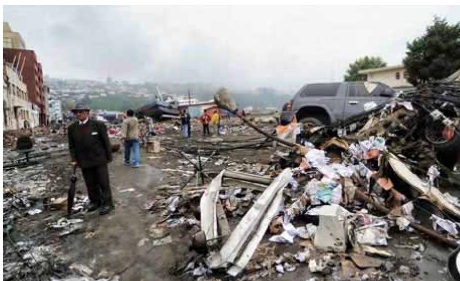
Figure 6.2 Photograph from cnn.com on February 27, 2010, Santiago damage
