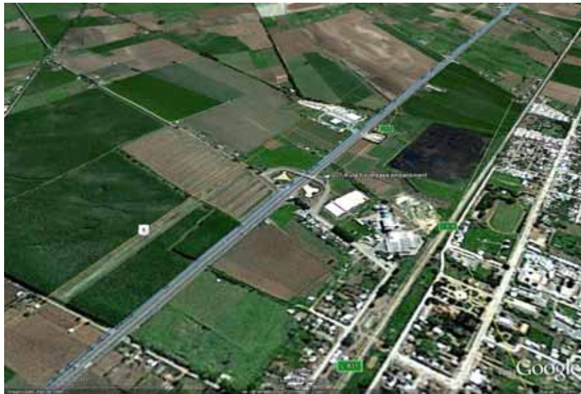
Figure 3.23 Route 5 South overpass embankment, looking north, to Retiro at Tucapel Mill (-36.051209°,-71.768005°)
