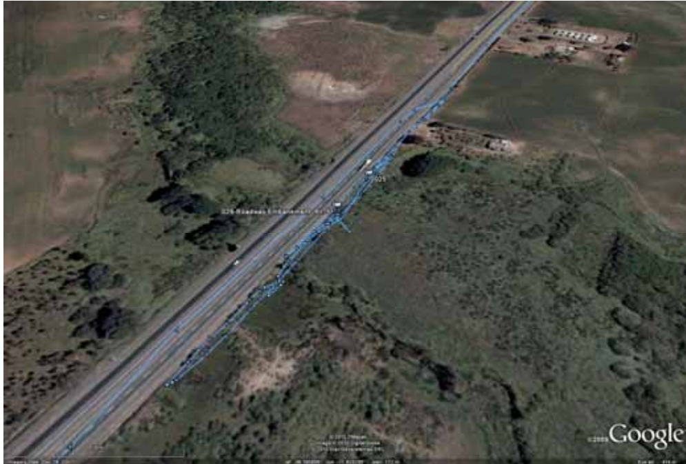
Figure 3.21 Roadway embankment ~5km south of Parral, north is up, Route 5 South (-36.185671°,-71.825415°)
