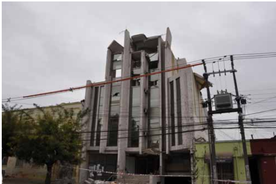
Figure 4.25 Edificio Aranjuez (6-story office building) was rendered nonfunctional due to nonstructural damage after the earthquake
