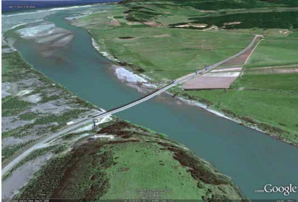
Figure 3.26 Puente Mataquito, looking north, April 16, 2010 (-35.050712°,-72.162258°)
