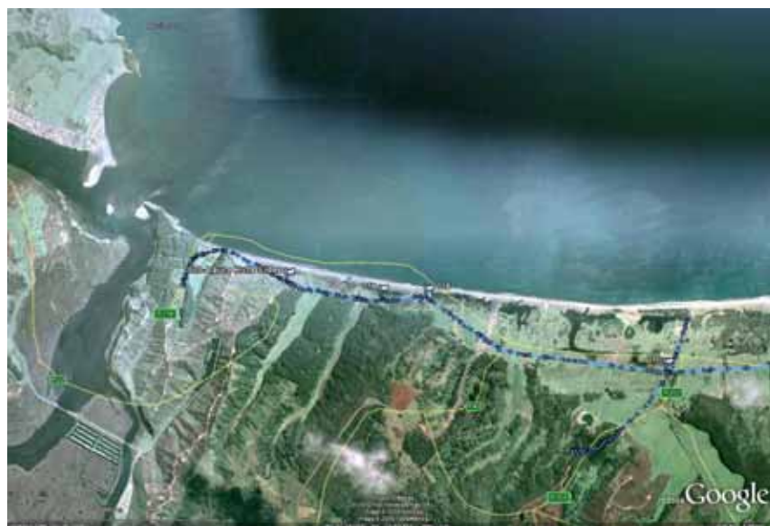
Figure 3.1 Arauco landslides/coastal bluff features view 1, (-37.246292°,-73.324251°) to (-37.242213°,-73.421207°)
