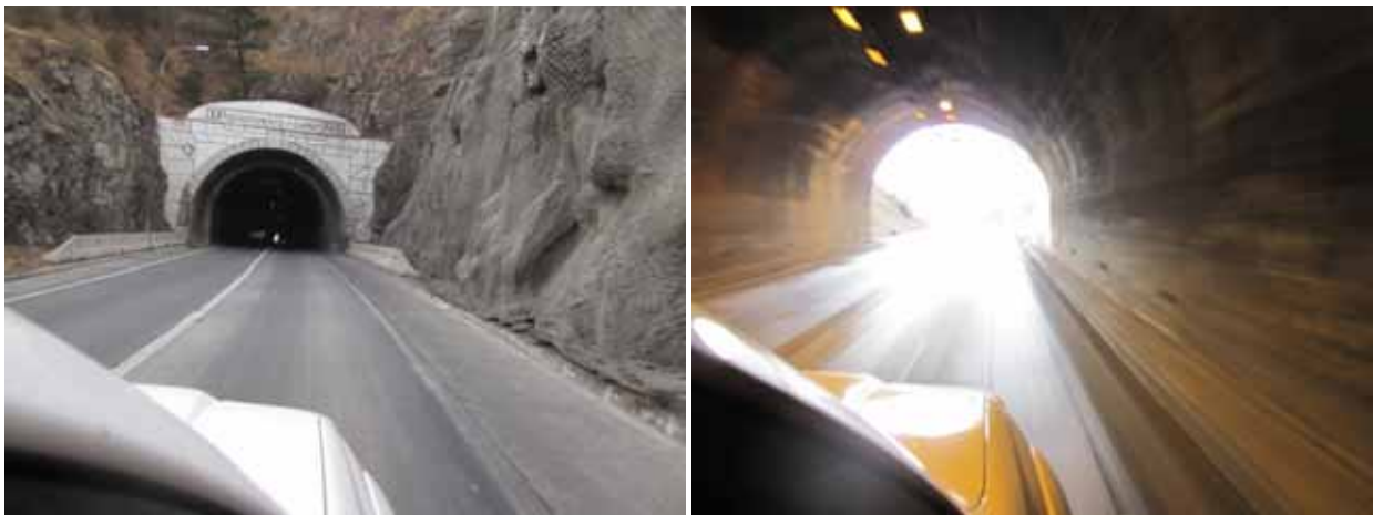
Figure 3.39 Highway tunnel, Route 5 South, April 12, 2010 (-33.912867°,-70.725533°)
