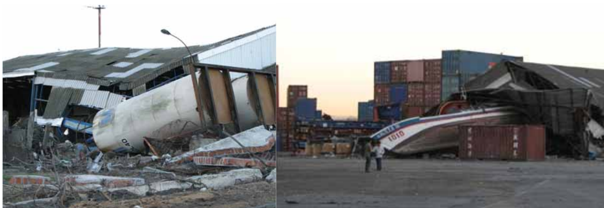
Figure 4.9 Effects of the tsunami on Talcahuano Bay. Top: toppled tank and collapsed building due to tsunami; Bottom: a dislocated ship, which damaged a storage building
