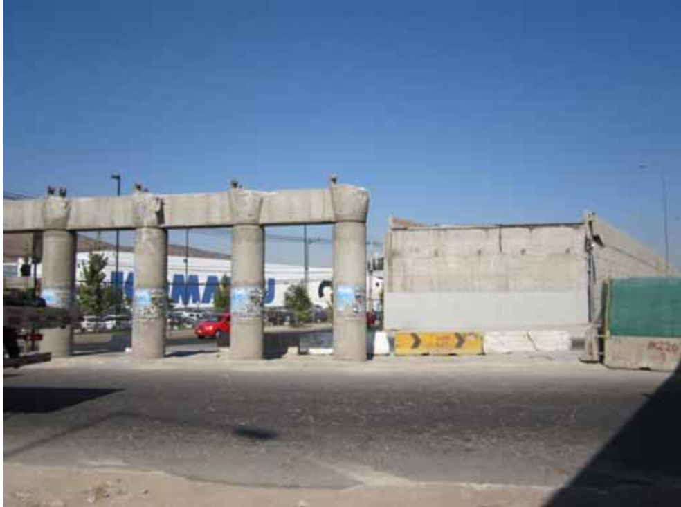
Figure 3.40 Mechanically stabilized earth wall, bridge ring 3, Lo Echevers Bridge, Santiago, April 13, 2010 (-33.376159°,-70.747742°)
