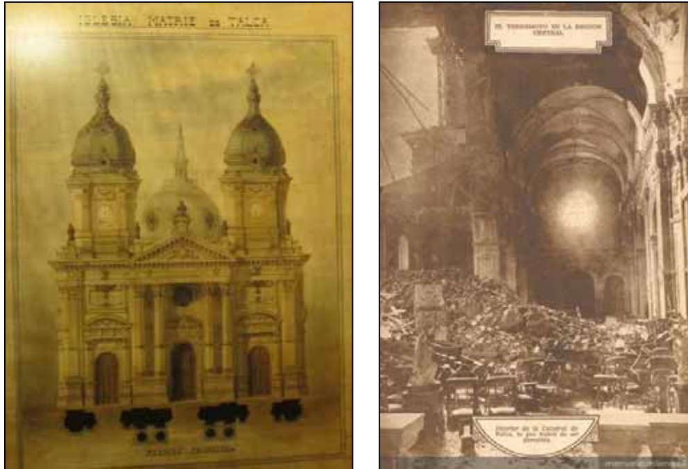
Figure 4.90 Cathedral of Talca before and after the earthquake in 1928
