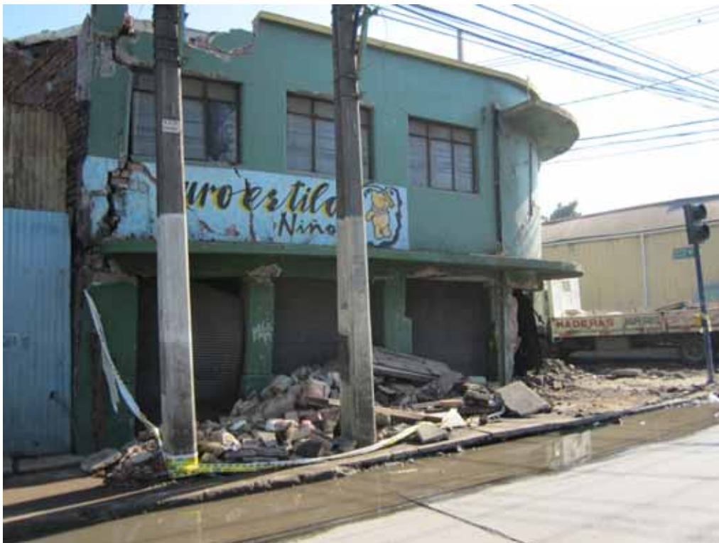
Figure 3.43 Tilting of the Green Building due to bearing soil failure, Talcahuano, April 15, 2010 (-36.714268°,-73.116368°)
