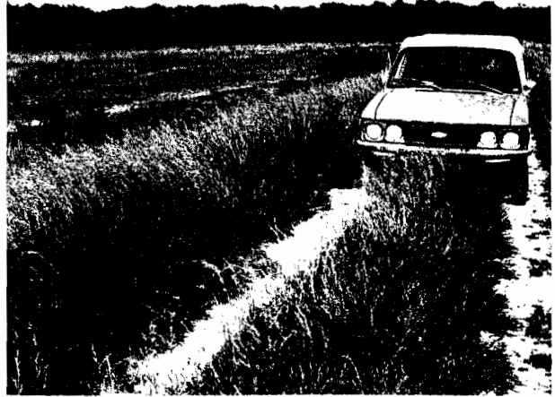
Fig. 2. Exterior levees constructed on Mingo National Wildlife Refuge have a top of at least 3 m with a slope of 3:1. These large levees readily support vehicles and heavy equipment and facilitate control of woody growth and muskrat damage.
