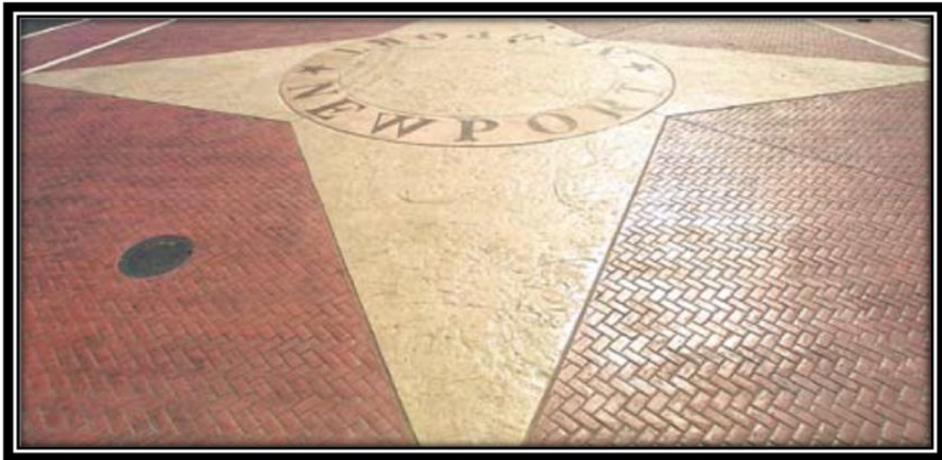
Figure 2.7 Brick pattern produced using a terra cotta color hardener and grey release while the star area was imprinted with a slate skin colored with buff hardener and grey release. Brass letters were embedded in plastic concrete (Boyer, 2007)
