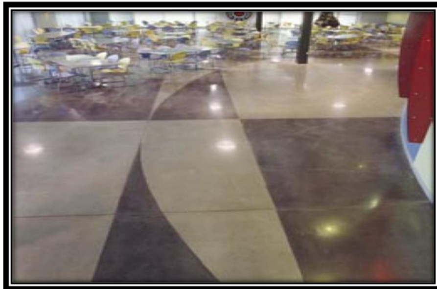
Figure 2.16 A cafeteria concrete floor that was saw-cut in a curved pattern followed by application of different colors of chemically reactive stains and finally polishing to give an attractive new look (Thome and Rizzo, 2004)
