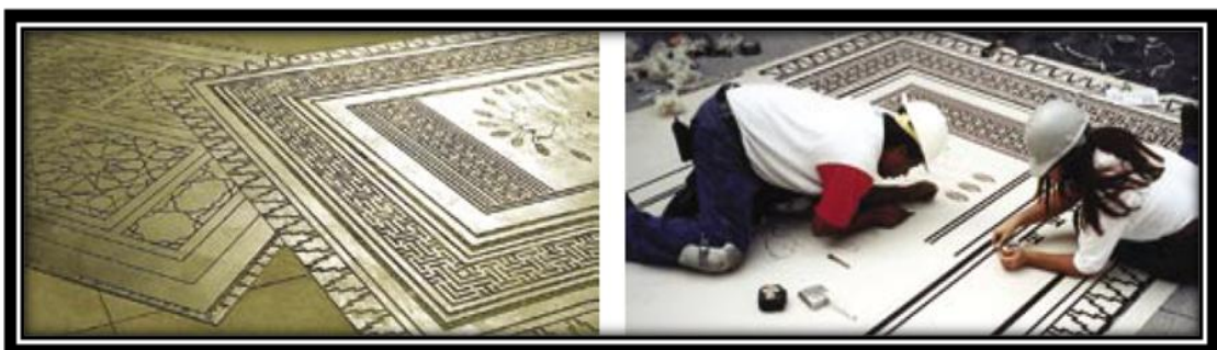
Figure 2.14 Removing parts of computer-cut template before sandblasting the floor for a final stunning look (Nasvik, 2004)
