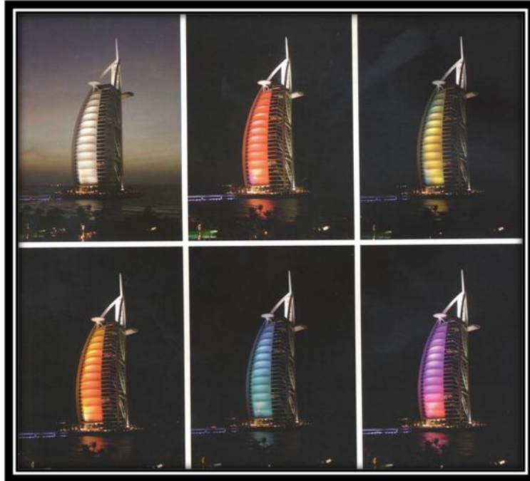
Figure 2.2 Computer-controlled color changing lighting concept at Burj Al Arab tower in Dubai (Porter and Mikellides, 2009)
