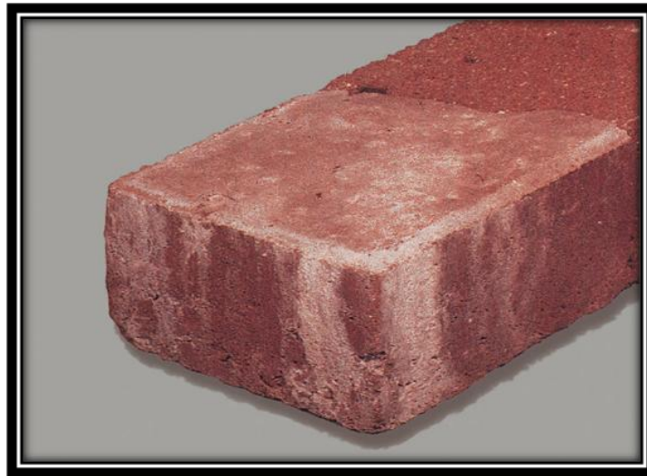
Figure 2.30 Effect of Efflorescence on Pigmented Concrete (Lanxess.com, 2013)
