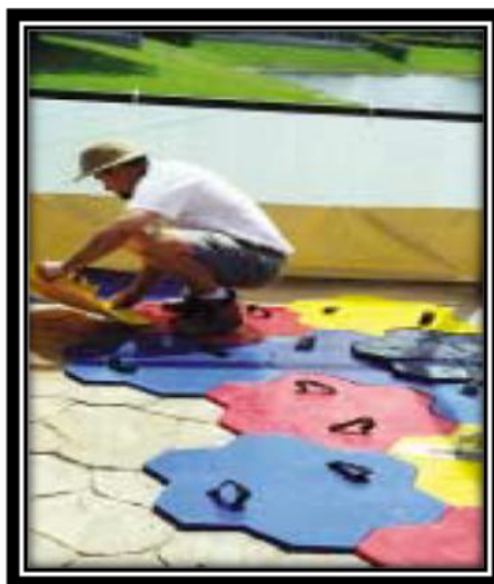
Figure 2.11 Stamping concrete patterns using a "walk-on" technique (Lamm, 2002)
