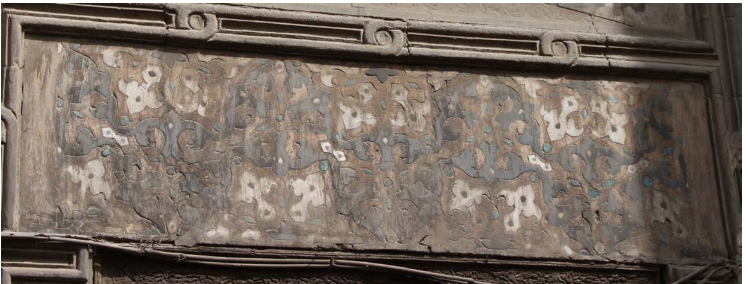
Fig. 4.39: Inlaid marble panel on the southwest side of the sabil
