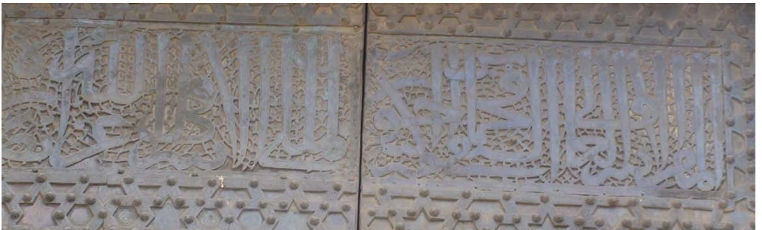
Fig. 4.6: The inscription on the upper band of the metal revetted door of the main portal
