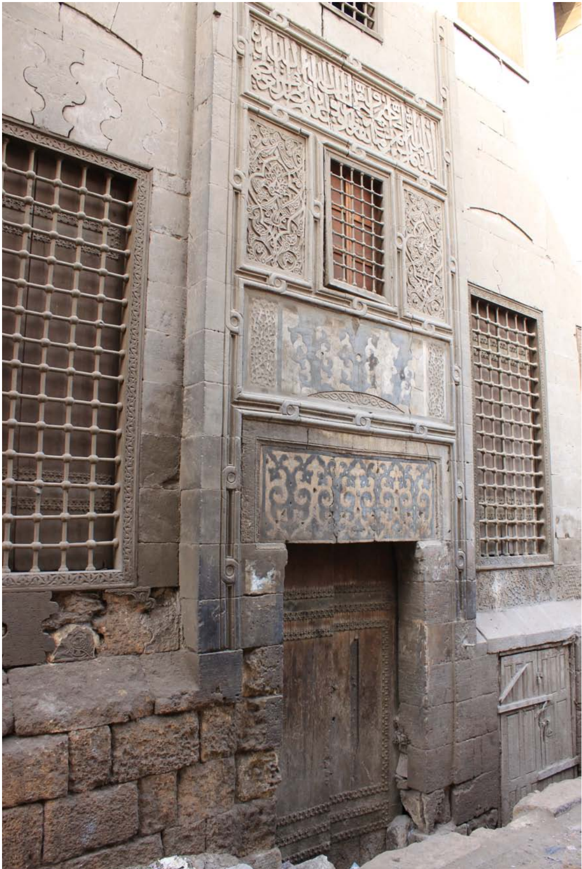
Fig. 2.14 Qibla façade portal leading to the mausoleum crypt
