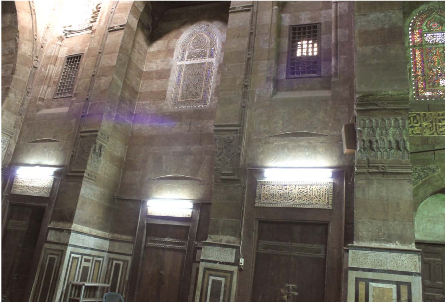
Fig. 4.25: Metal band doors of the interior
