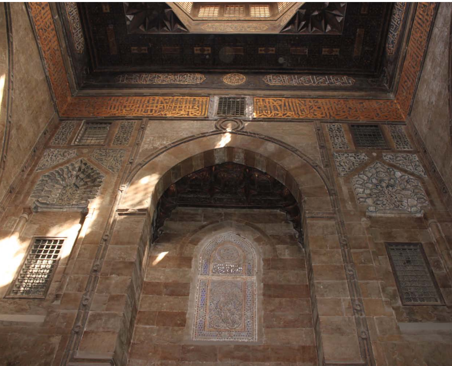
Fig. 2.16: Windows of the cells above the southern lateral iwan
