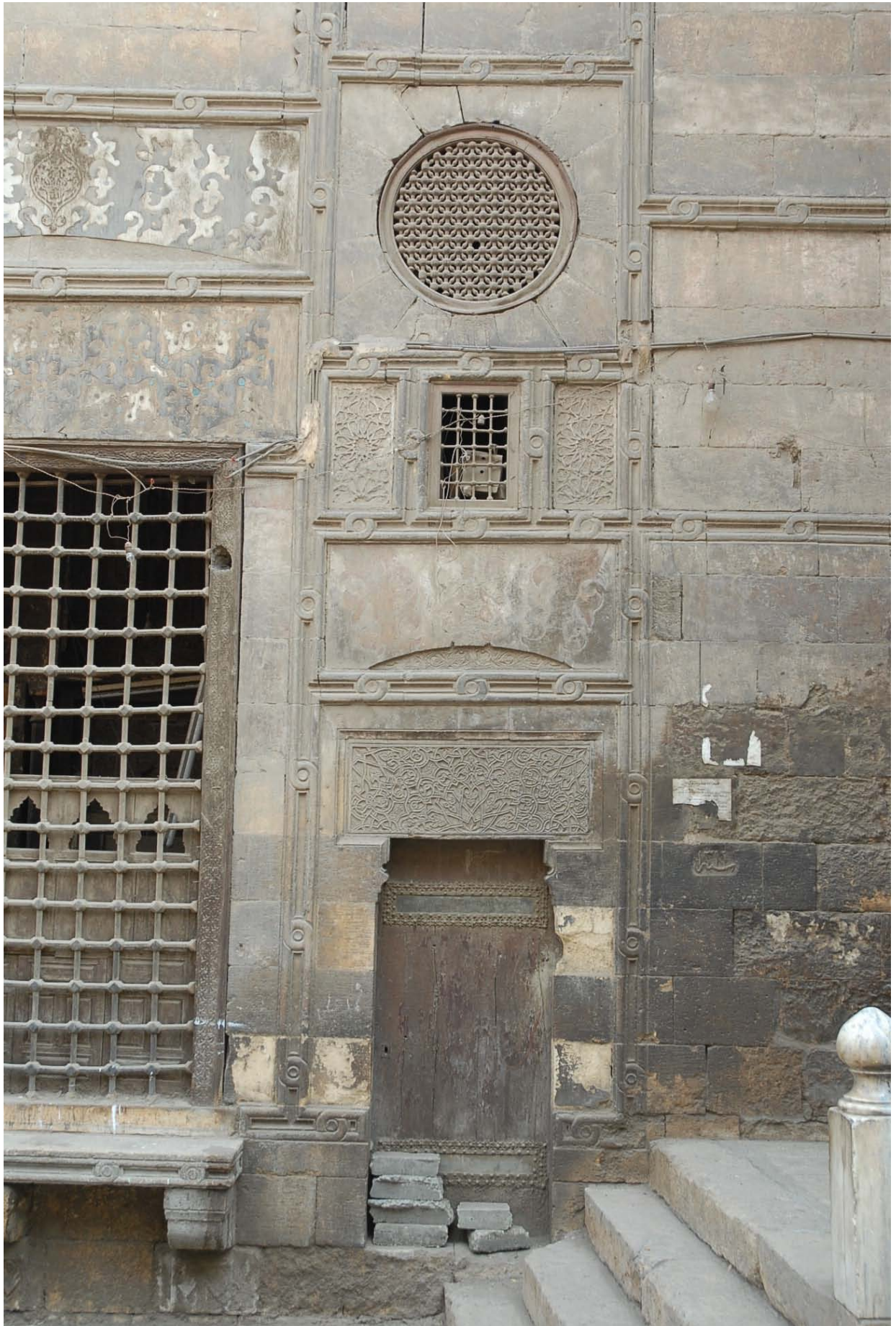
Fig. 2.9: Door of the sabil on the southwest facade
