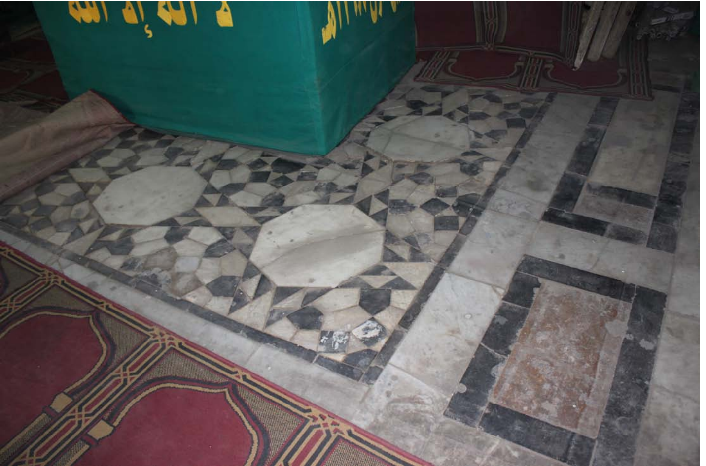
Fig. 4.32: The inlaid marble floor of the mausoleum
