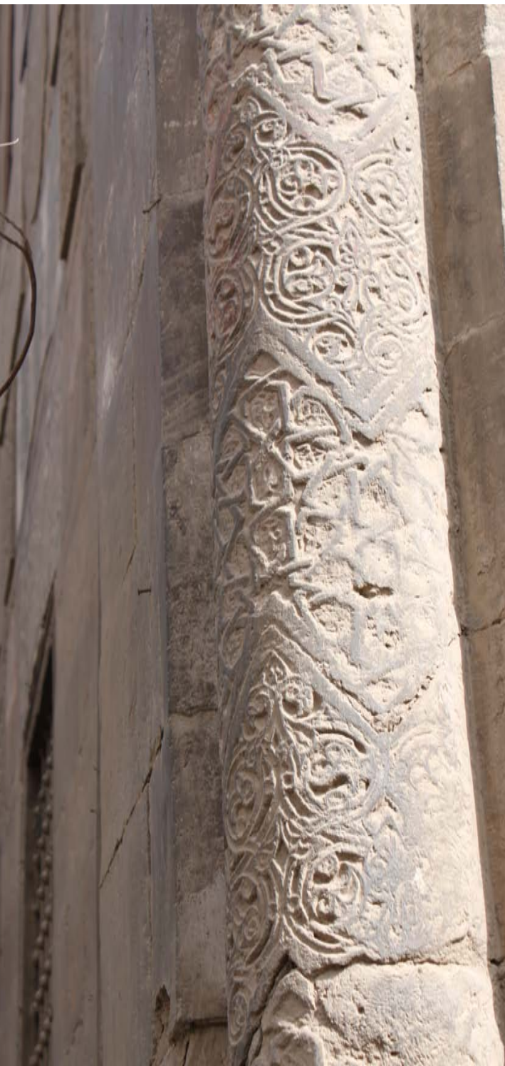
Fig. 4.33: Engaged column of the northwest façade
