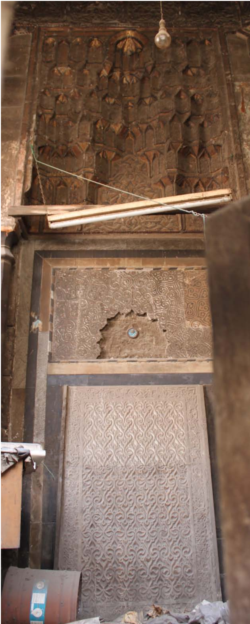
Fig. 2.10: The shadirwan of the sabil with its muqarnas hood
