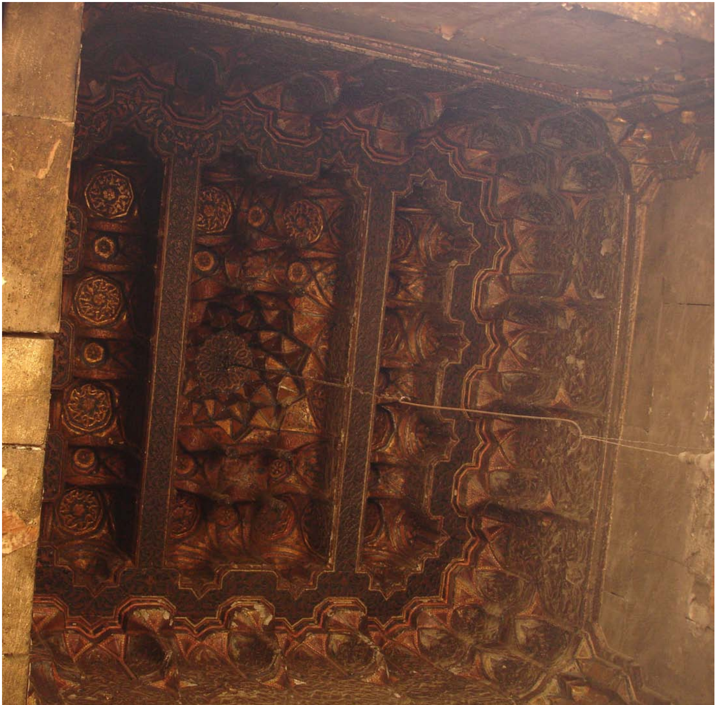
Fig. 2.11: The ceiling of the sabil
