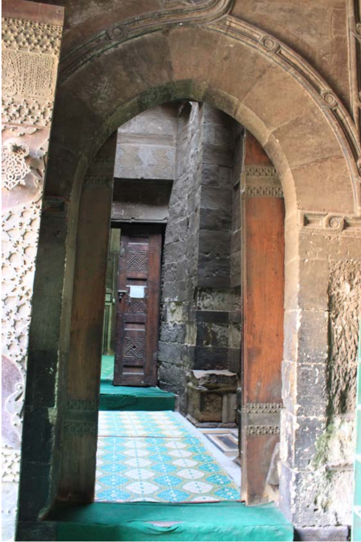
Fig. 3.4: The sliding door leading from the entrance vestibule to the sahn of the mosque of Qijmas
