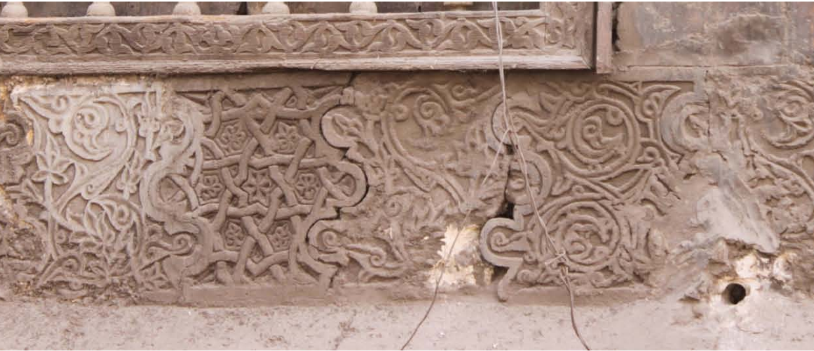
Fig. 4.35: Carved horizontal panel on the northwest façade
