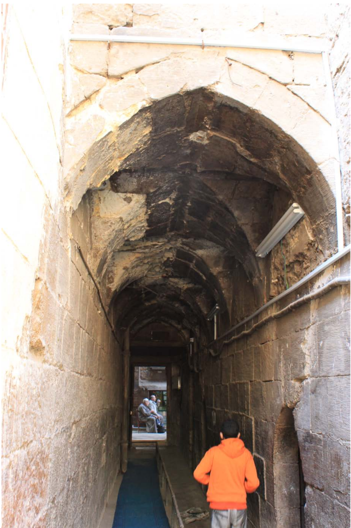
Fig. 2.19: The groin vaulted corridor of the ablution court
