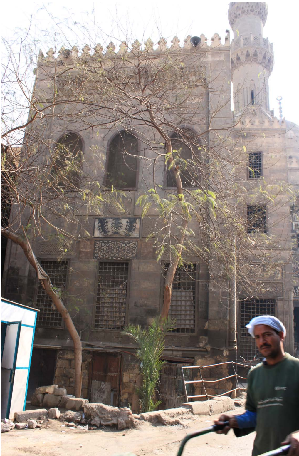
Fig. 2.6: The northwest facade
