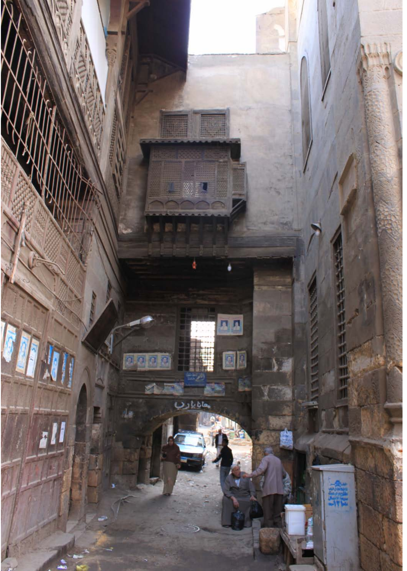
Fig. 2.18: The bridge leading to the mosque's dependencies
