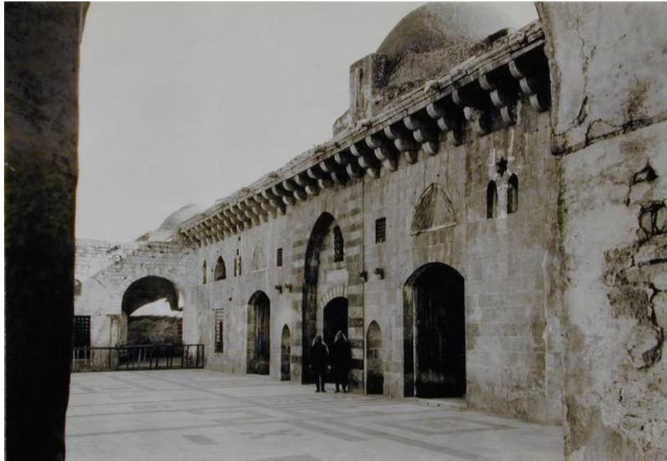
Figure 31. Courtyard of the mosque of Hama (from http://archnet.org/library/sites/one-site.jsp?site_id=7999 )
