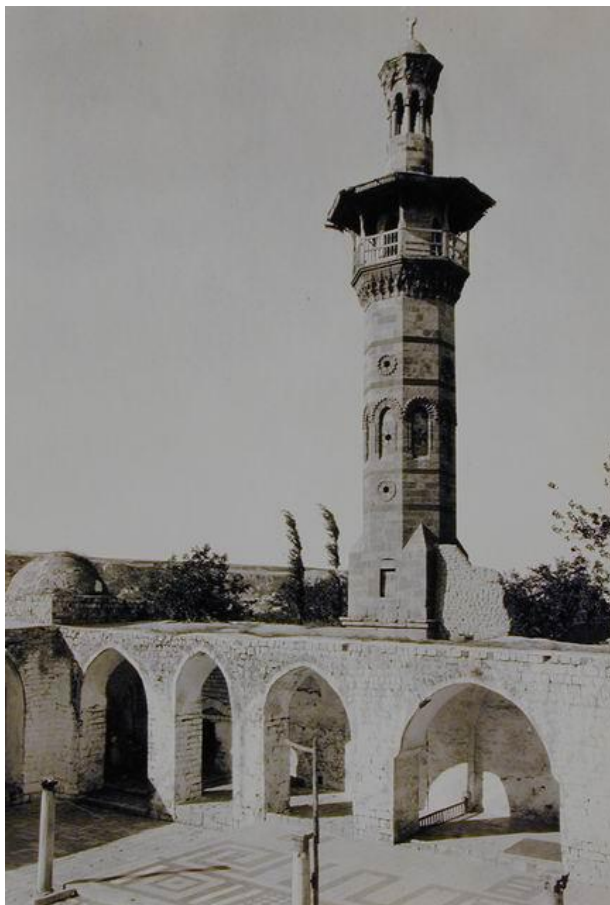
Figure 32. Riwaq of the mosque of Hama (from http://archnet.org/library/sites/one-site.jsp?site_id=7999 )
