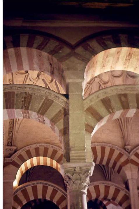
Figure 41. The double tiered arches, Cordoba mosque, an influence of the Great Mosque of Damascus (from http://archnet.org/library/sites/one-site.jsp?site_id=31 )
