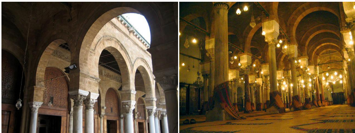
Figures 36- 37. Horseshoe arches in the mosque of Zaytuna, similar to Cordoba mosque (from http://archnet.org/library/sites/one-site.jsp?site_id=14061 )
