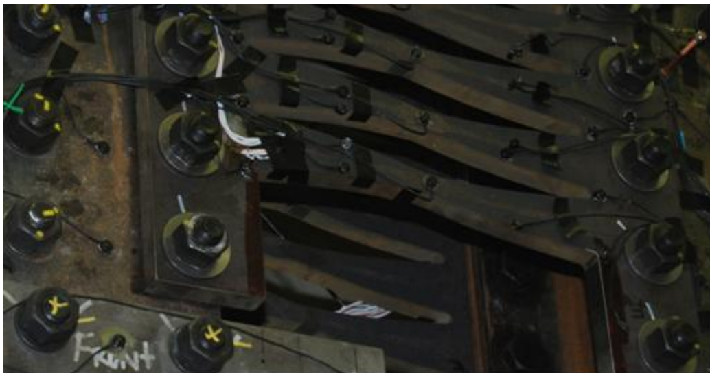
Figure 5.30 Photograph of Fuse Showing Slip Relative to the Column and Yielding Along the Fuse Links for Specimen A4
