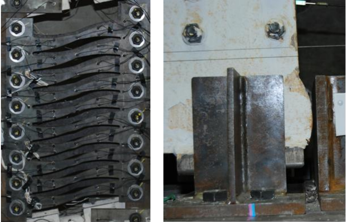
Figure 5.16 Photograph of the Deformed Specimen A2 Fuse (Left) and Uplifted Column Base (Right)
