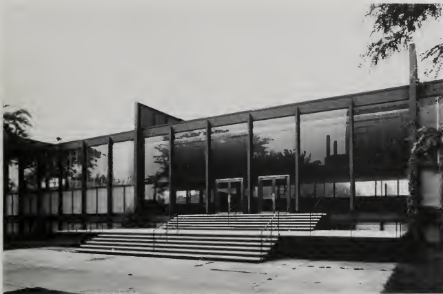
Ludwig Mies van der Rohe, Crown Hall, Illinois Institute of Technology, Chicago, 1952–56 (photo: Botond Bognar).
