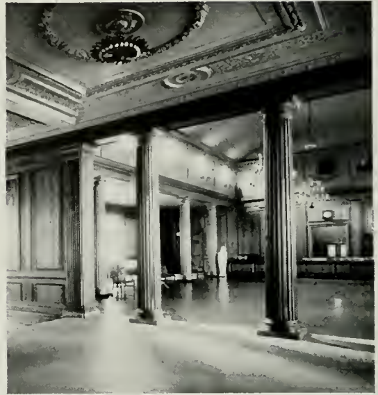
Inside the main library when constructed. Soon we will see the interior of the new Natural Resources Building.
