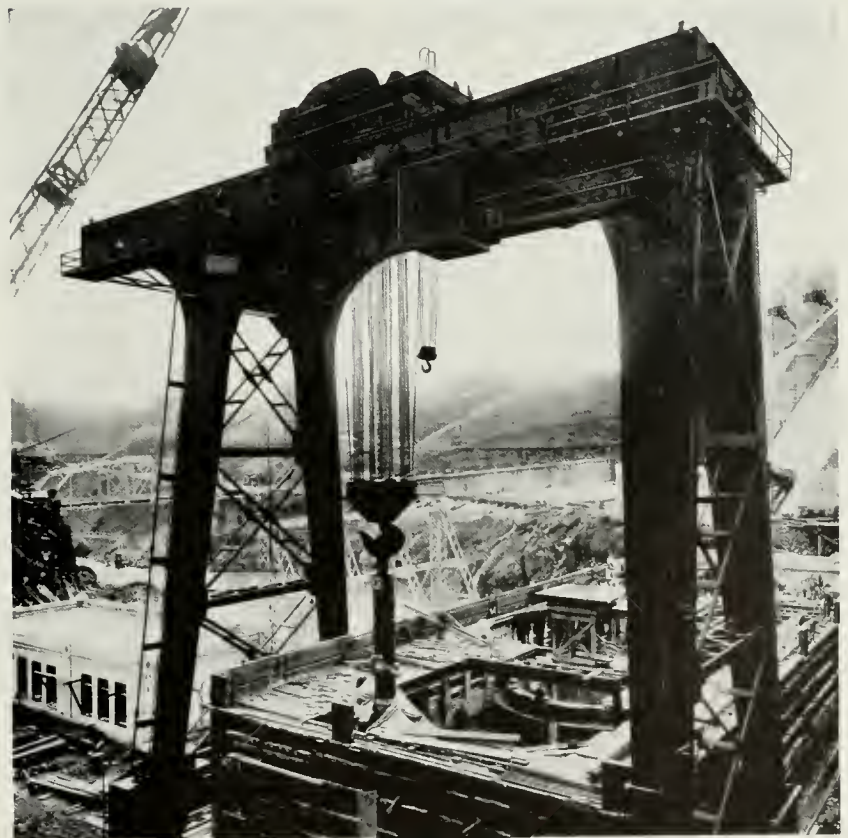
BUILD OUTSIDE when your crane is too large to fit inside the building. That's what they did for the gantry-crane erected at Ariel Dam power house in Washington state.
