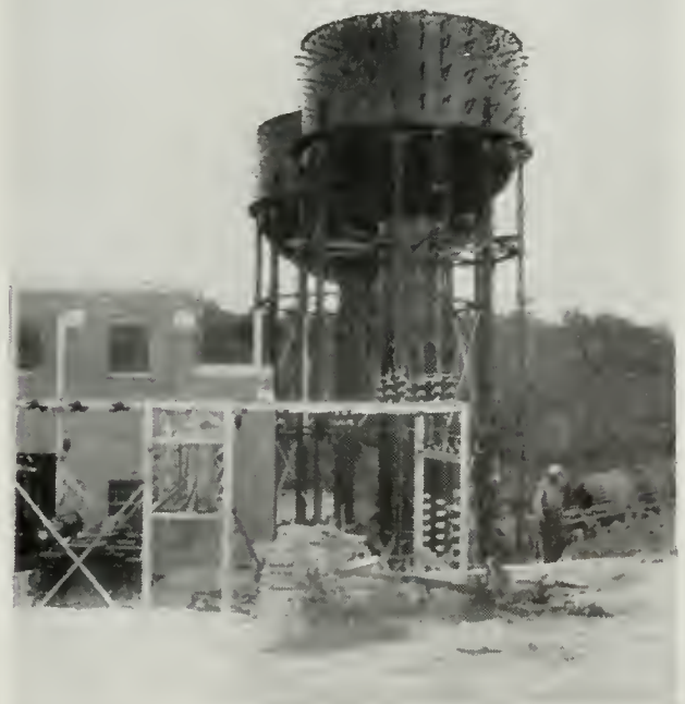
Power House and Surge Tanks
