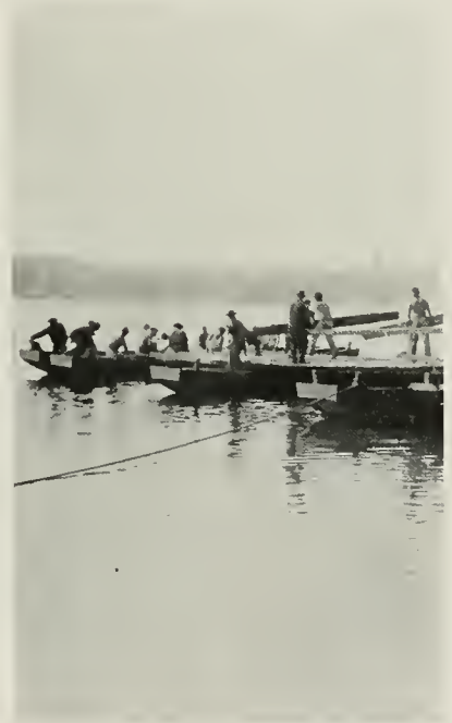
Pontoon Bridge Construction
