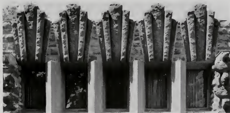
Cover: The Joshua Melson House by Walter Burley Griffin, 1912, Rock Crest Development, Mason City, Iowa Detail of second-story windows. The five-part keystones are actually monolithic blocks of reinforced concrete. Photographs of Mati Maldre
