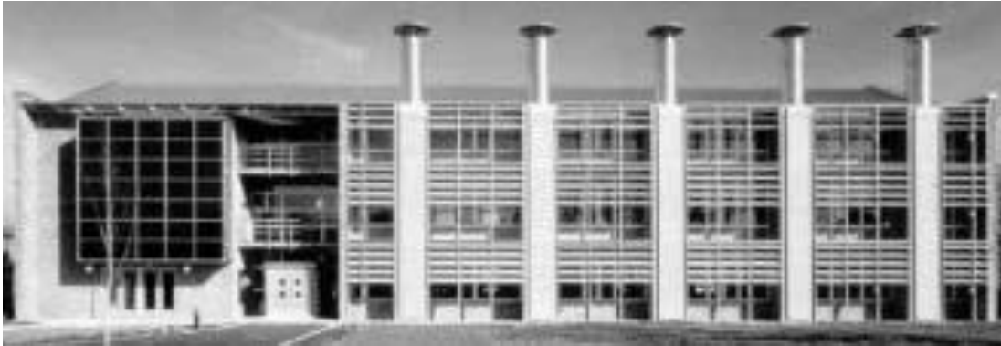
Figure 2.7 The BRE building with chimneys extending well above roof level to increase the stack potential and achieve stable wind-induced suction
