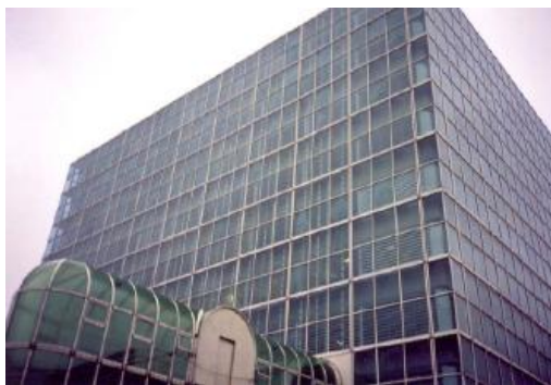
Figure 3.15 Occidental Chemical Building, southwest corner
