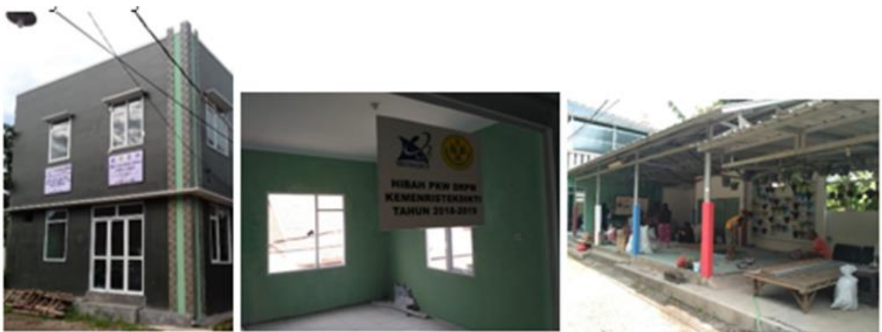
Figure 5. Construction of a waste bank building
