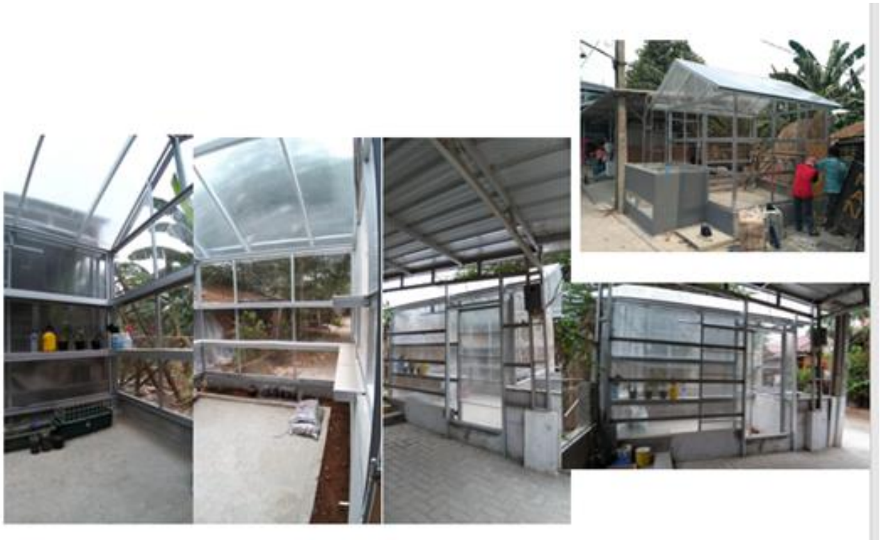
Figure 7. Construction of a greenhouse and composter
