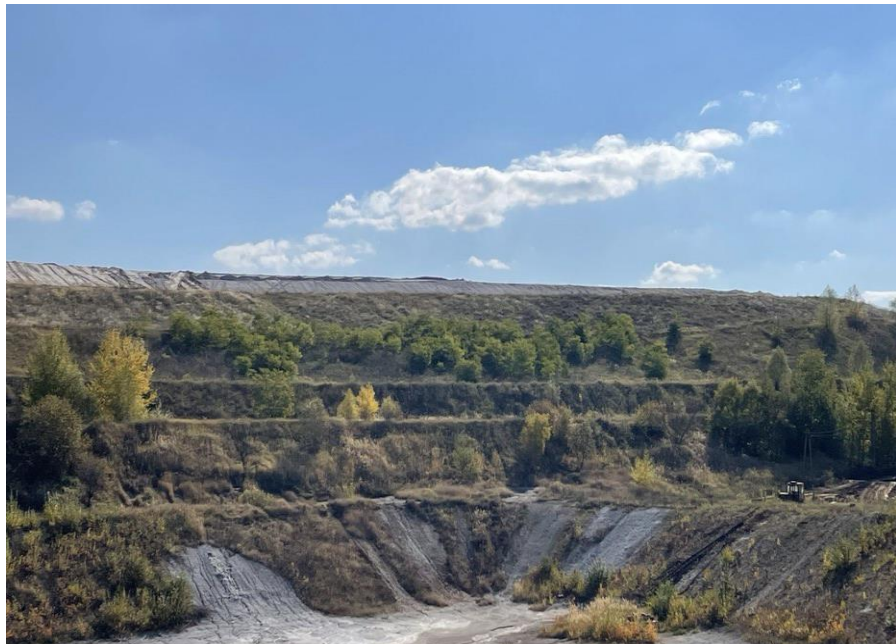
Figure 1.5 – Phosphogypsum terraces from the southeast side of dump, Sumy Region (Ukraine), 2021
