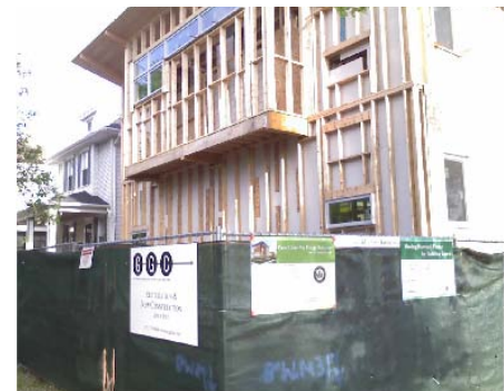
Yannell House - Cook County
