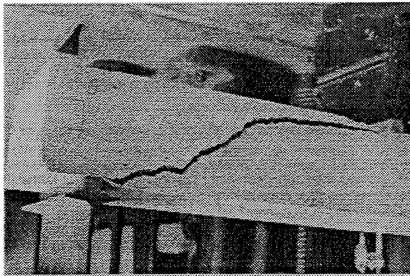
Fig. 8.32 Diagonal Tension Shear Failure in Reinforced Concrete Beam (from [56])
