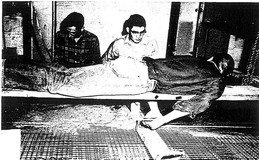
(a) Placement of Wire Reinforcement
