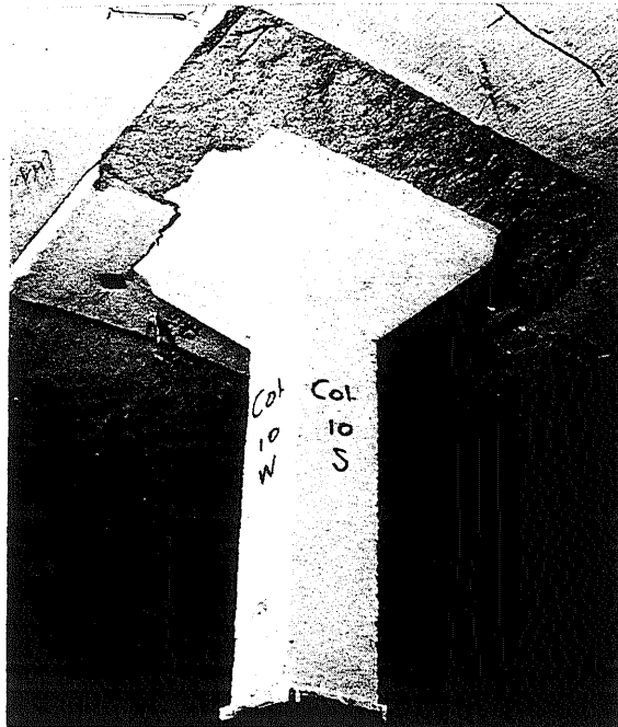
(a) View from Southwest
