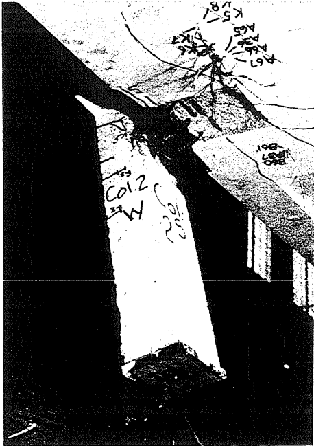
(a) Column 2 After Failure
