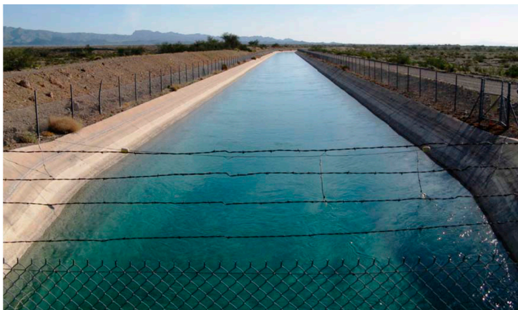
Figure 2. Canal in the Mojave Desert of California showing wildlife-proof protective fencing along the edges. Photo taken from a road across the canal.
