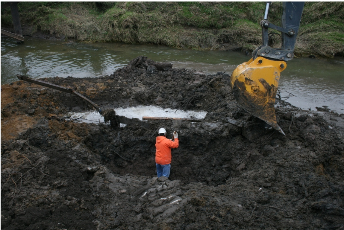
Figure A-13. Earth dike surrounding embedded piles.
