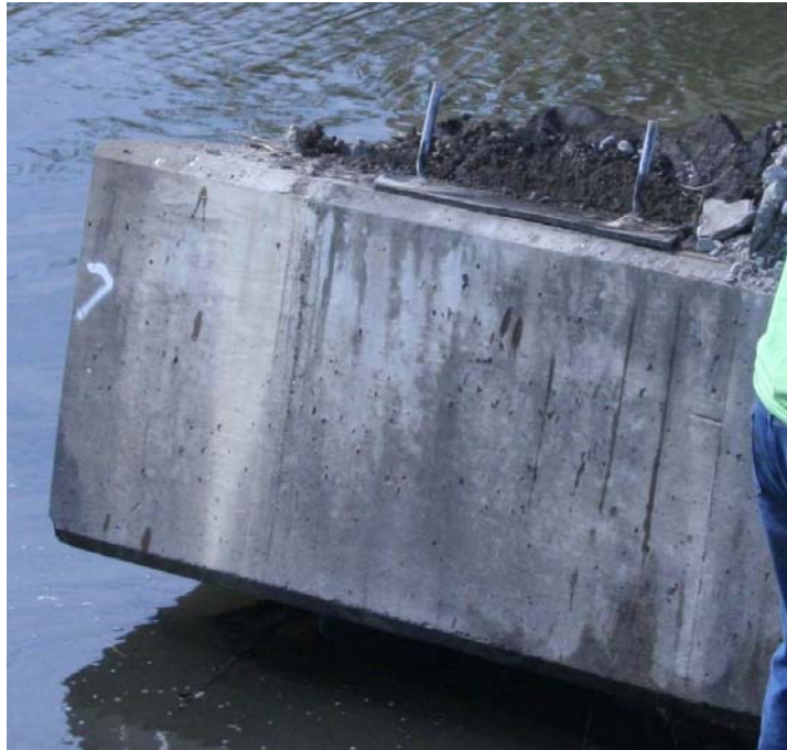
Figure A-3. 3/4 inch steel dowels.
