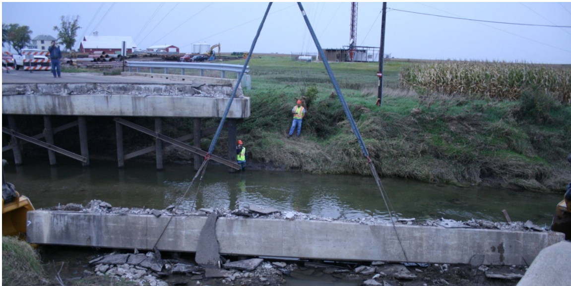
Figure A-6. Bent 3 pile cap attached to crane and excavators.
