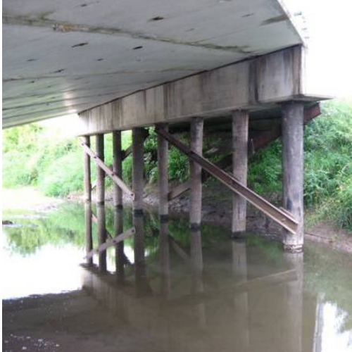
Figure 3. Midspan bent 2 timber pile foundation.
