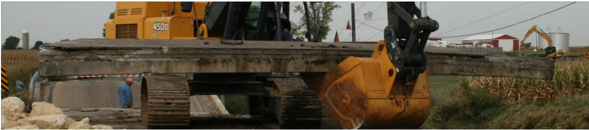
Figure A-4. Extracted deck beam.
