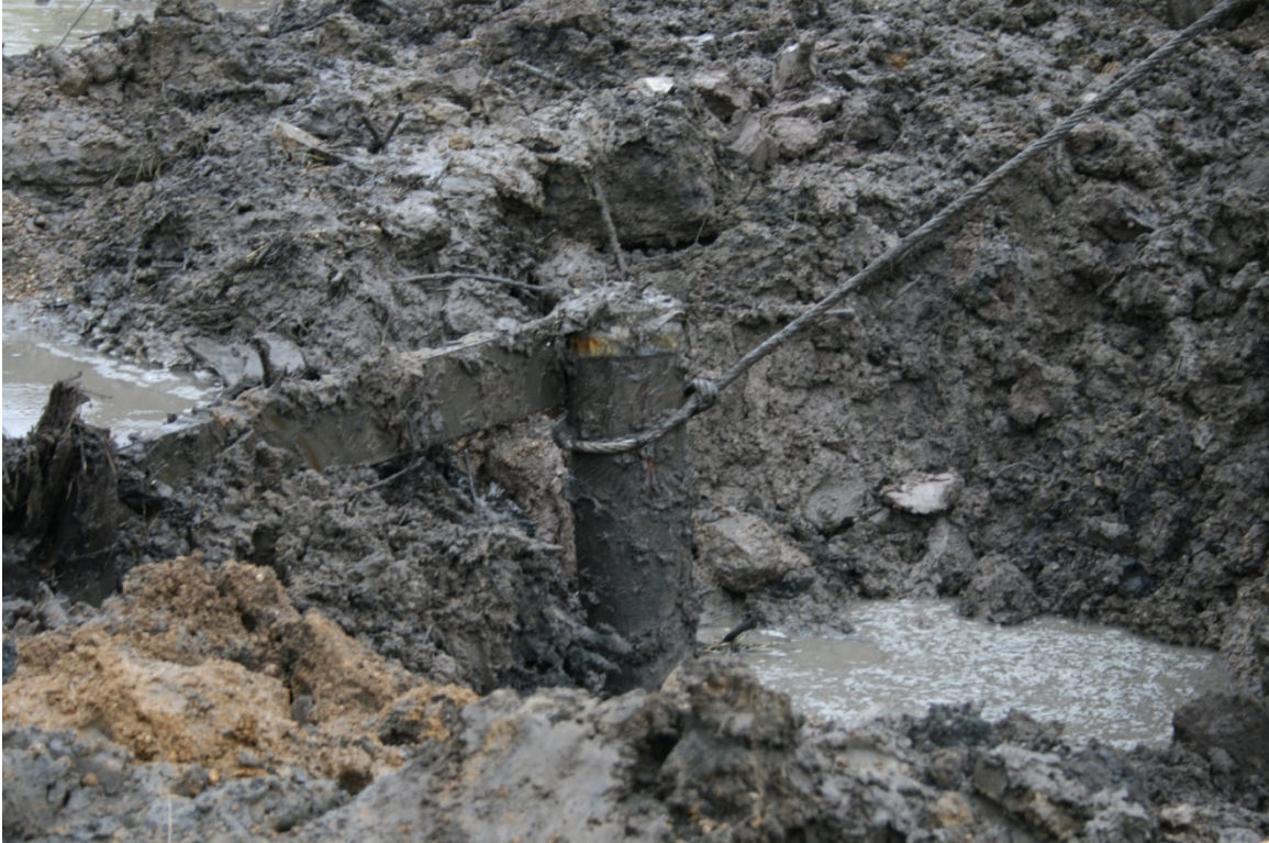
Figure A-14. Extraction of post of pile 1.
