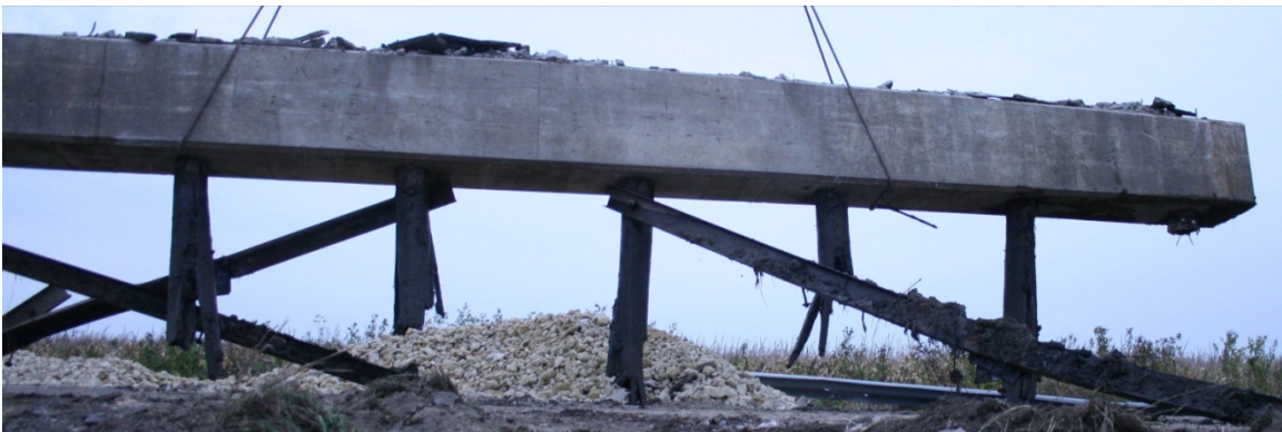
Figure A-9. Extracted pile cap.
