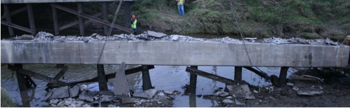
Figure A-7. Bent 3 pile cap partially removed from riverbed.
