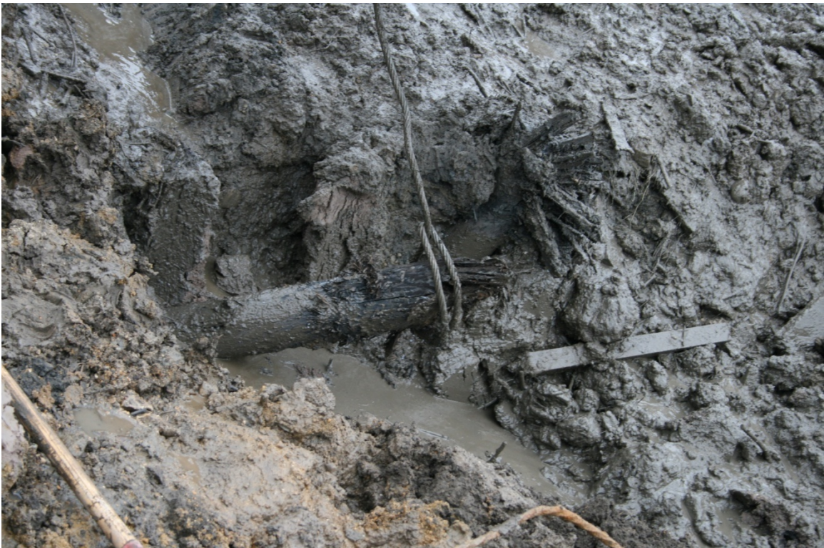
Figure A-15. Failure of embedded pile 1 under applied lateral load.
