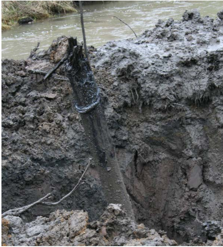
Figure A-16. Extraction of pile 2.
