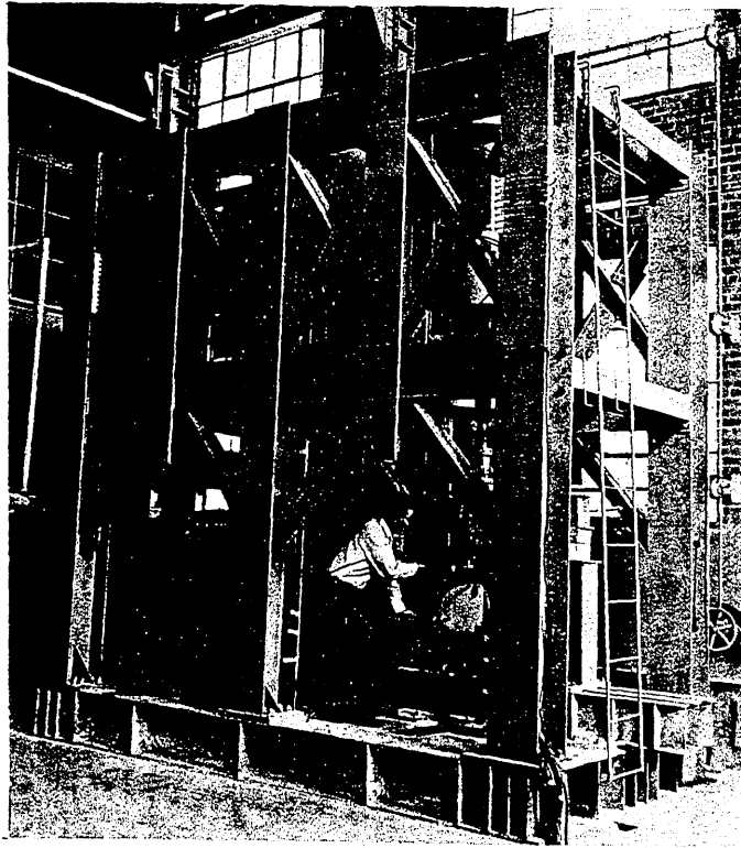
(a) Test Frame
