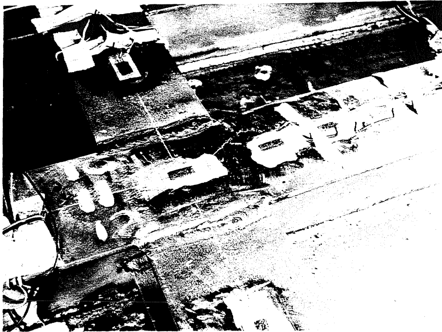
FIG. 5.2.1 FAILURE OF WELD BETWEEN LONGITUDINAL AND TRANSVERSE BEAMS IN SPECIMEN V-F, ~130-KIP LOAD
