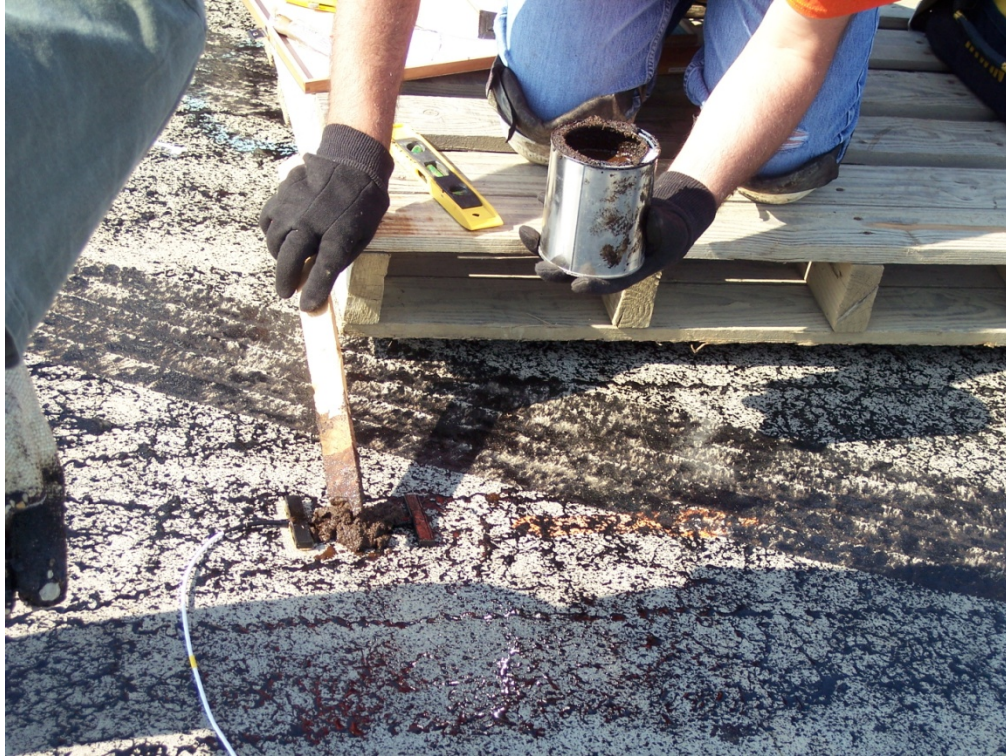
Figure 5-8. Covering the strain gauge with emulsified asphalt sand.
