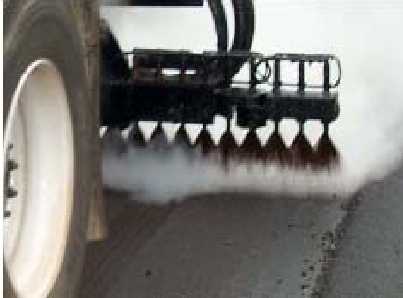
Figure 3-6. Proper overlap and spray bar height (WSDOT, 2003).
