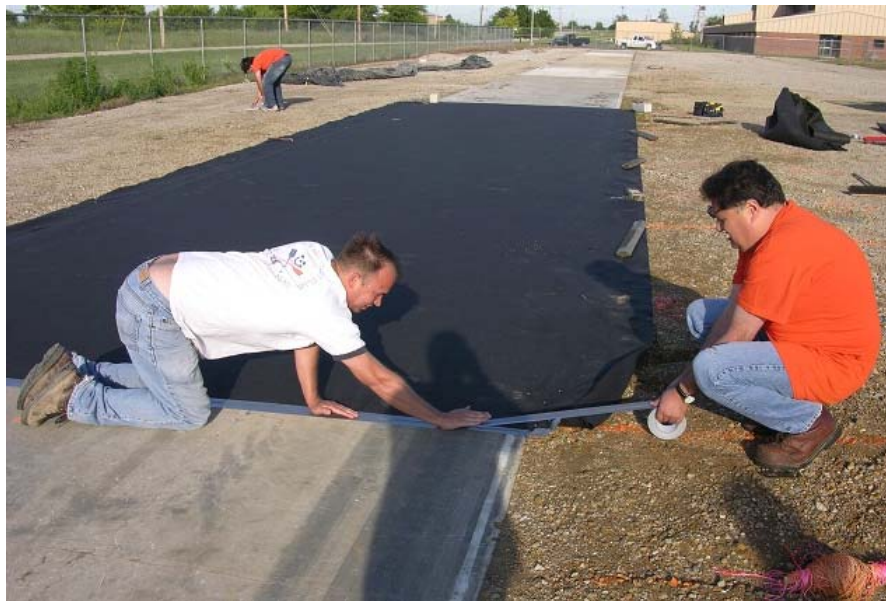
Figure 4-3. PCC surface protection with geotextile sheet.
