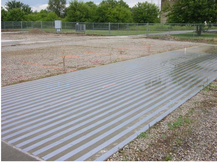
Figure 3-8. Preparation for zebra sections with duct tape on PCC surface.
