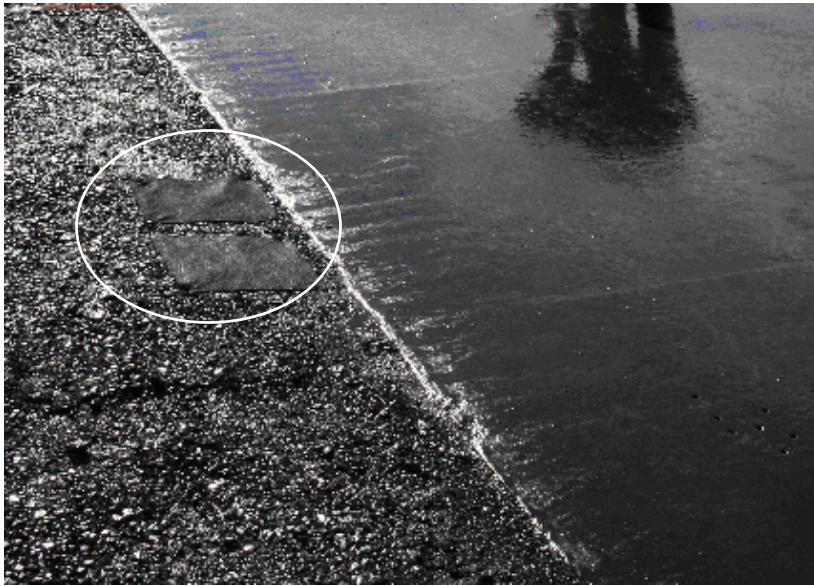
Figure 4-2. Tack coat application rate verification with geotextile pads.
