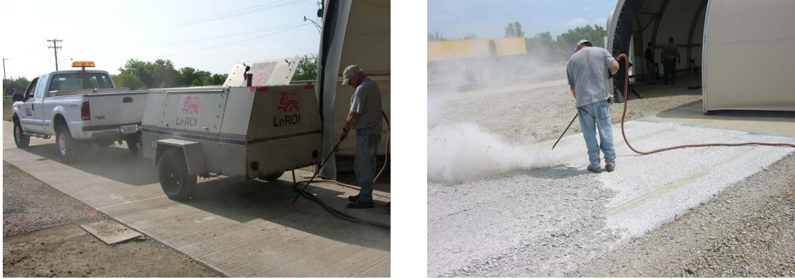
Figure 3-4. PCC surface cleaning with air blast.
