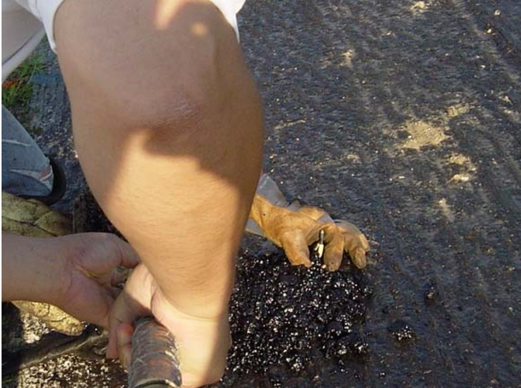
Figure 5-12. Surrounding the thermocouple with HMA.
