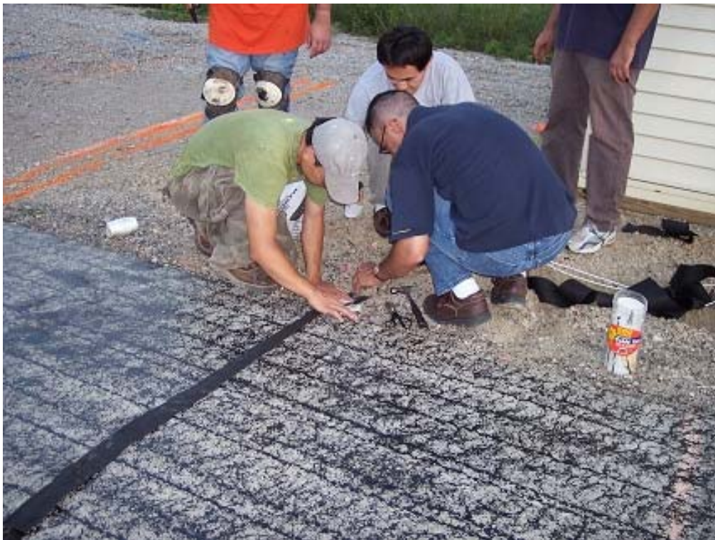
Figure 5-9. Protecting strain gauges with geosynthetic fabric
