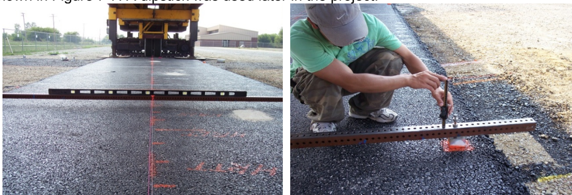
Figure 7-7. HMA overlay surface profile measurement in ATLAS Test 3.
