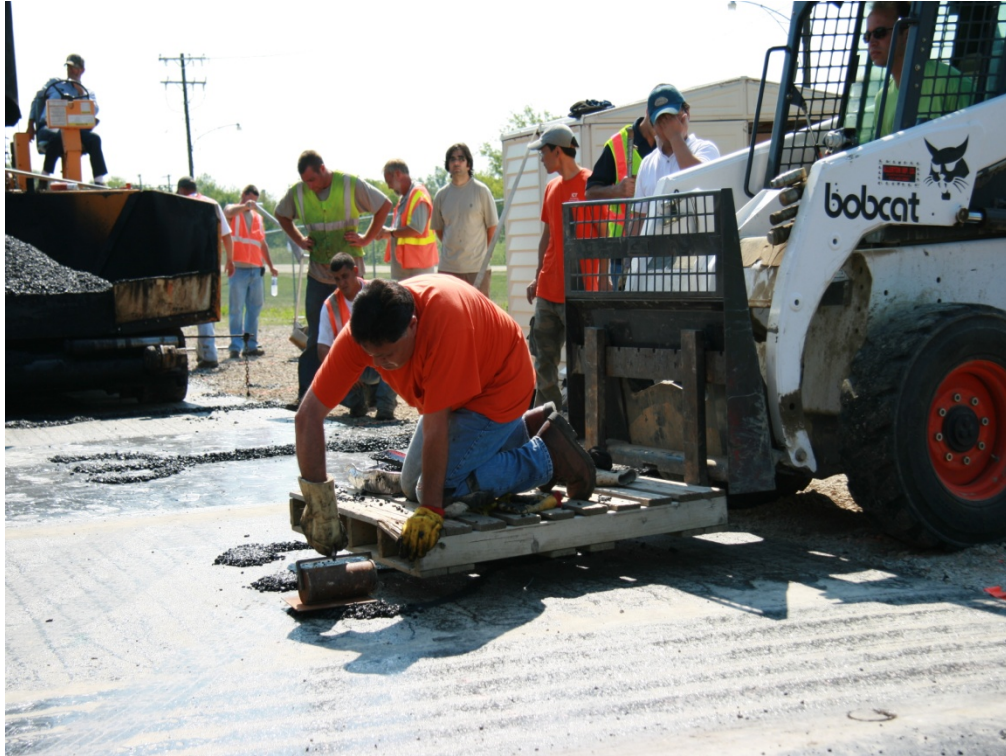
Figure 5-10. Rolling and compacting HMA sampled from paver over the strain gauge.
