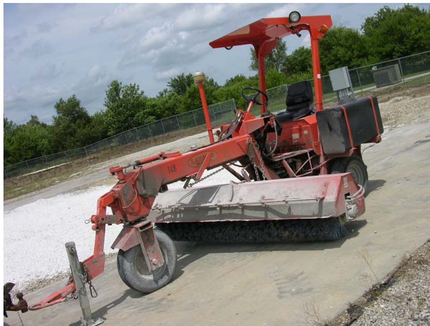
Figure 3-5. Powered-broom for cleaning milled sections.
