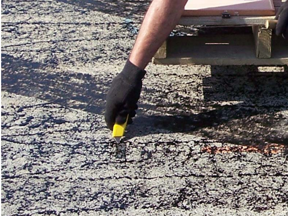
Figure 5-6. Removal of duct tape for gluing the strain gauge end.
