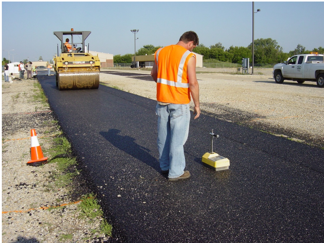
Figure 6-2. Density check by using a nuclear density gauge.
