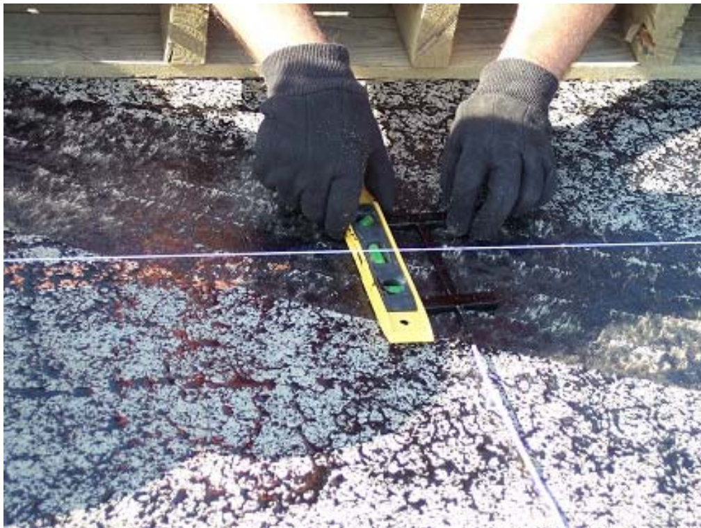
Figure 5-7. Maintaining leveled strain gauge by use of a bubble level.
