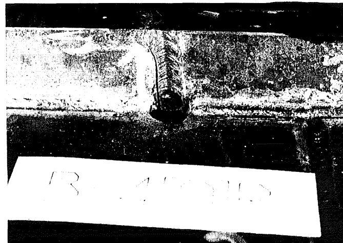
b. SPECIMEN B-4(O)R : FAILURE IN BUTT WELD
