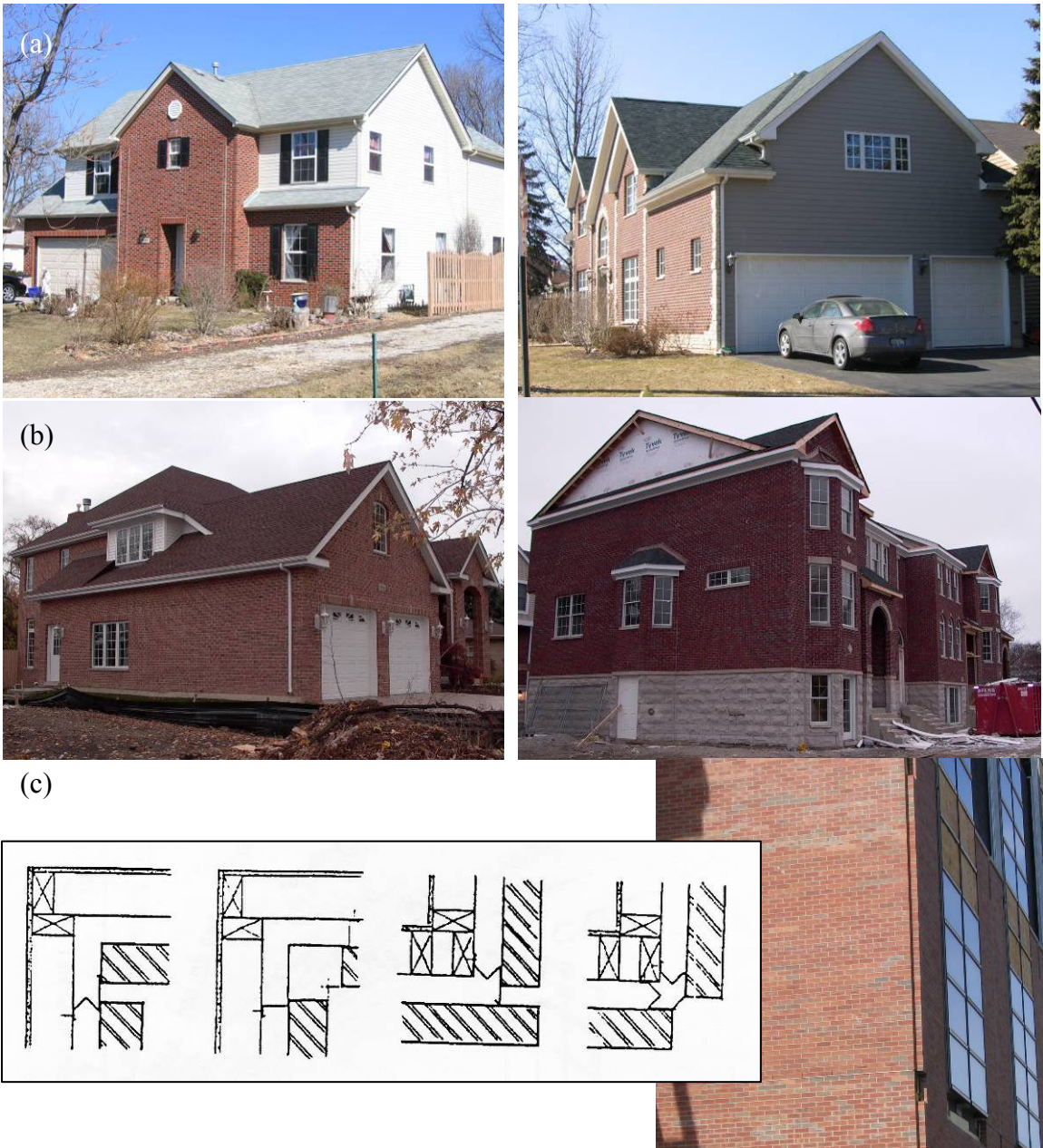
Figure 1.3 – Typical architectural styles for brick veneer construction: (a) front wall only brick veneer, (b) continuous around corners and multi-story brick veneer, and (c) expansion joint (open) wall corner details (corner detail sketches from Lapish (1988)).
