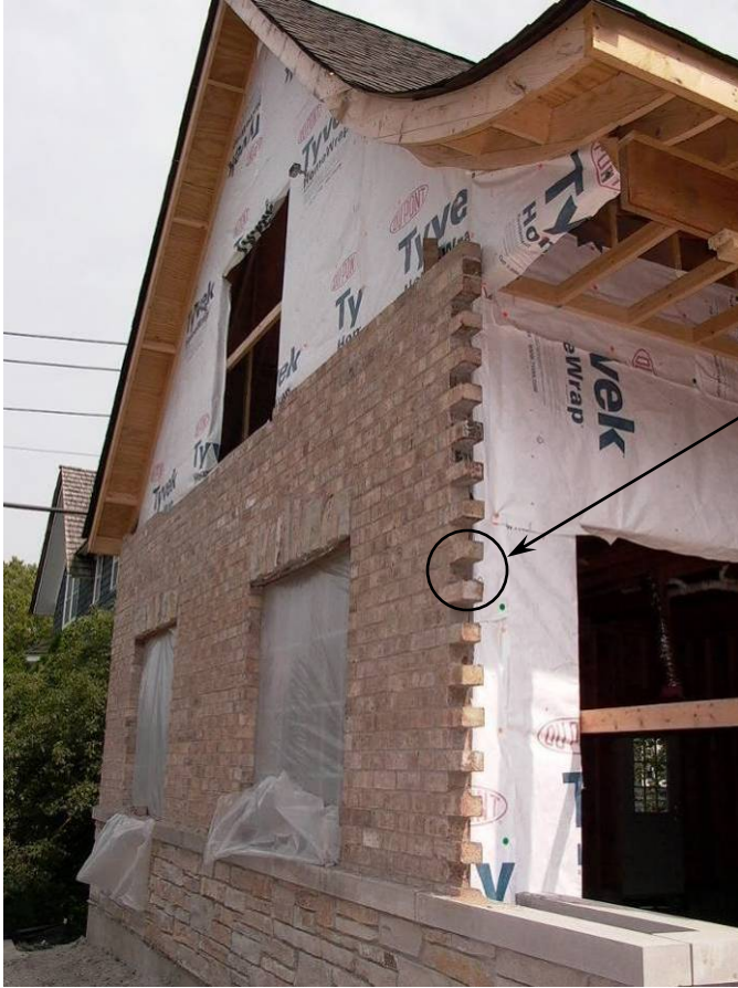
Figure 2.1 – Residential brick veneer home during construction, with excessive mortar droppings in the wall cavity.
