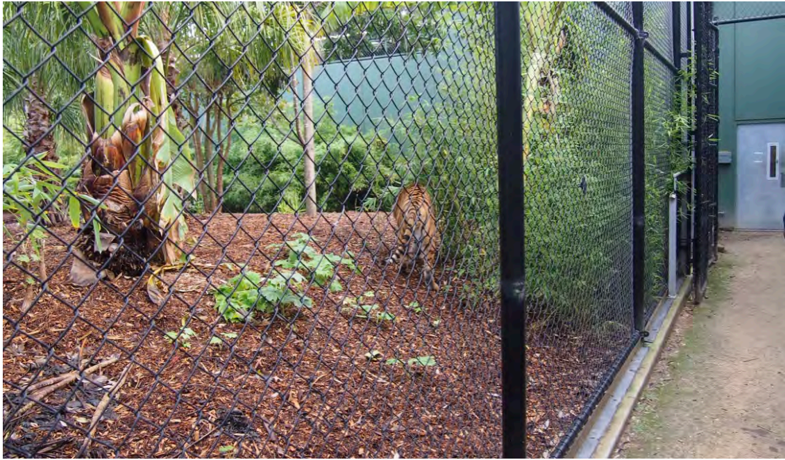
Image 37: Malleable mesh to stop the Sumatran Tigers from climbing. The foldout access point is visible in the third panel. This is also the Watch where you step enclosure.
