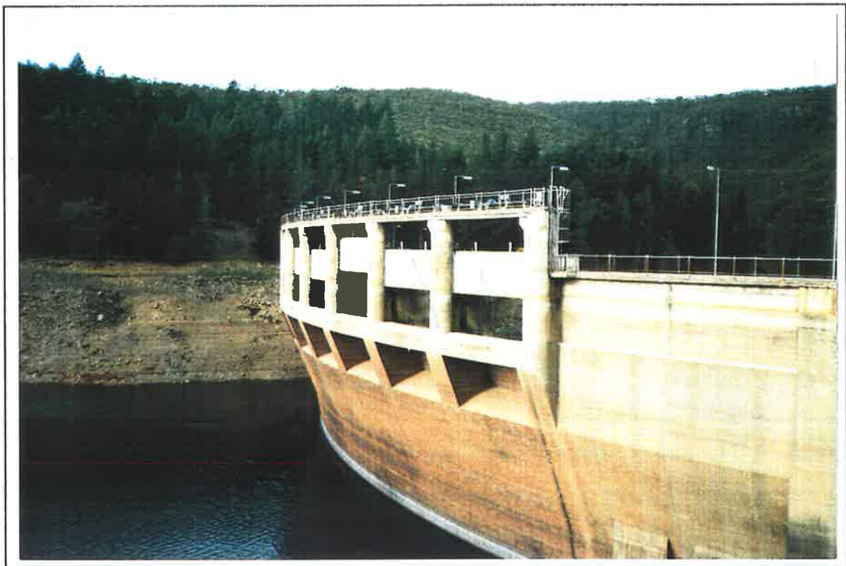
Figure 4.2 Mt Bold Reservoir with Gates set to Maximum Openings (August 1992)
