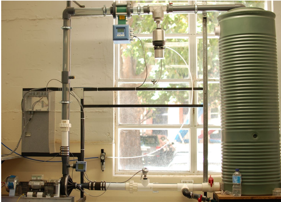
FIGURE 6.2: Pump test system. The pump is connected to a closed loop system of piping with a reservoir tank. At the top of the system is an electromagnetic flow meter followed by a computer controlled process control valve.
