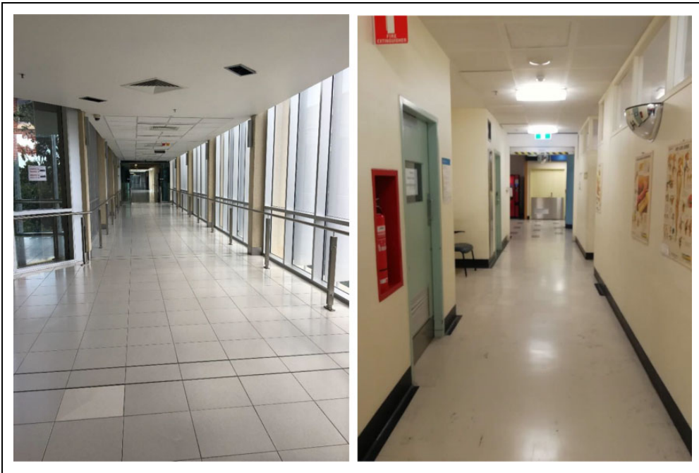
Figure 2. Differences in lighting in the corridors of the new sections of the hospital (photo on the left, Hospital Street, first floor) and old area of the hospital (photo on the right, Outpatients building corridor, ground floor).
