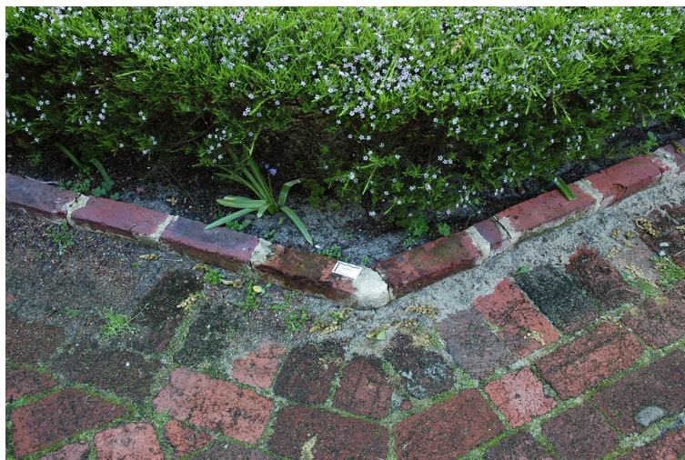
Fig. 4. Photograph of manufactured earth materials comprising brick paving, mortar (mixture of cement, fine sand and lime) and adjacent transported organic-rich garden soil (modified from Raven et al. 2019 ).
