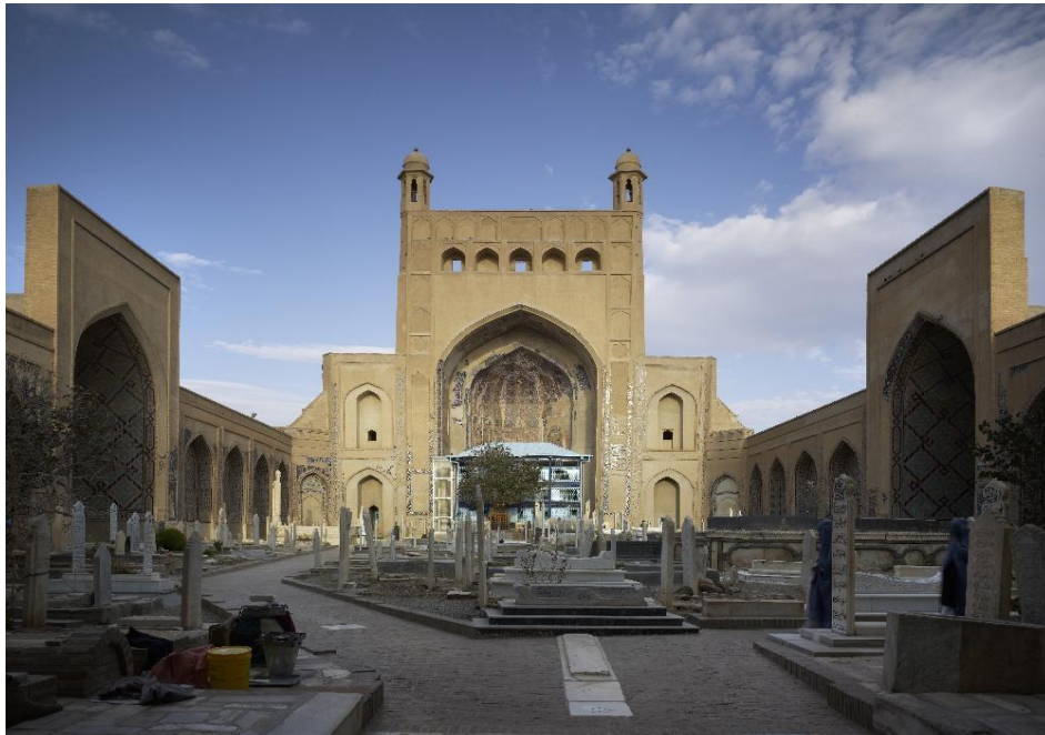
Figure 2-8. The internal courtyard of the shrine complex of Khāwja ‘Abdullāh Ansārī in Gāzurgāh, north-east of Herat, today Afghanistan (Source: https://archnet.org , Aga Khan Historic Cities Programme)
