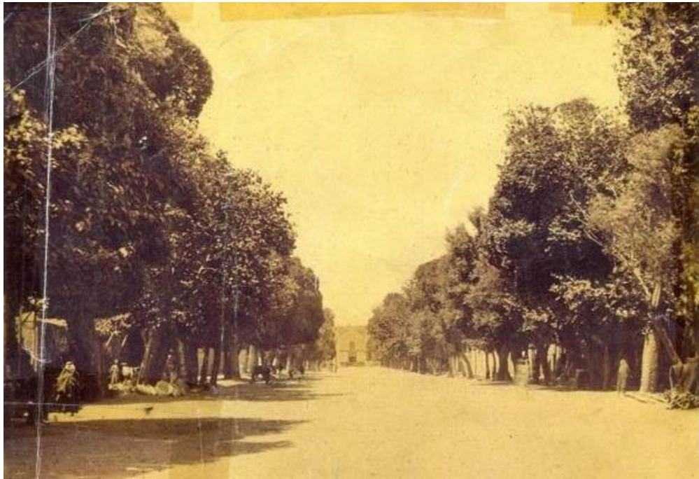
Figure 6-7. Khayābān in Qazvin and the ‘Āli Qāpū gate, 1921 (Source: http://traffic.qazvin.ir )
